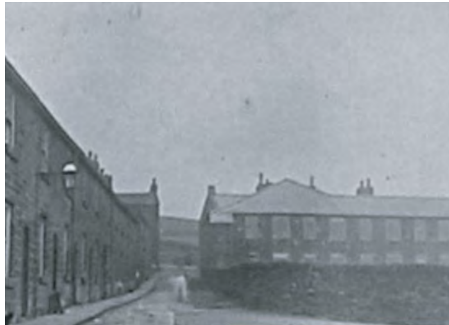
Figure 6: Early 20th century photograph of Mount Pleasant showing the mill building to the right which has since been replaced by 1980's infill development
