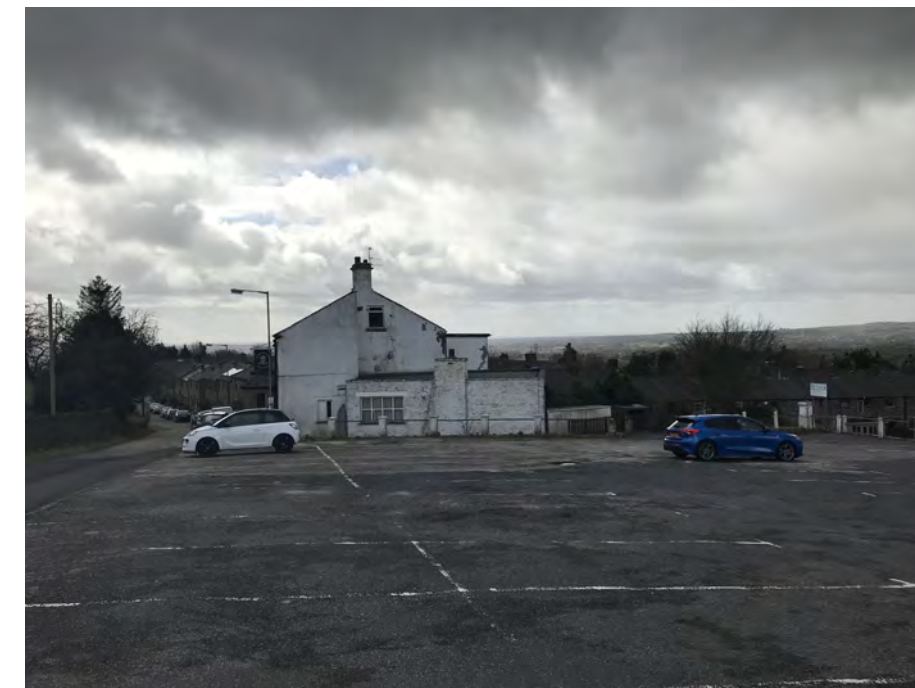
Figure 3: Northern elevation of Lord Raglan Public House and car park
