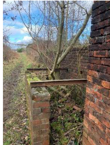
Figure 14 – A possible old tank base on the side of a derelict outbuilding in the central south west of site.
