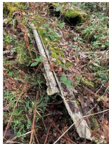
Figure 18 – A pile of suspected ACM on site.
