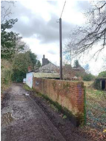
Figure 1 – Looking east from the north west of site showing the north western site boundary with an overhead electric cable supplying the site.
