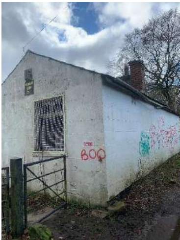
Figure 3 – The bungalow in the north west of site.
