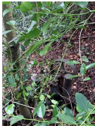
Figure 24 – The cast iron pump on the north western bank of the pond.
