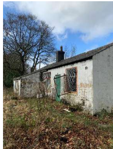
Figure 22 – The bungalow in the north west of site.
