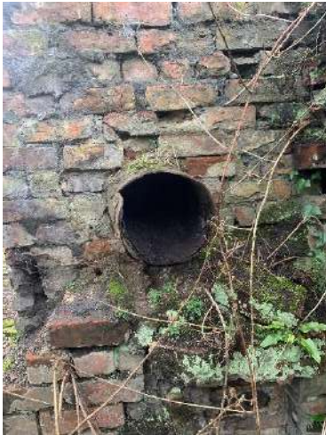
Figure 13 – The inlet at the base of the chimney.
