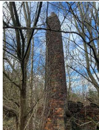
Figure 12 – The c. 15.00m tall chimney in the central south west of site.
