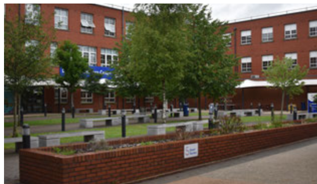
3.59 North Wing south elevation and East Wing west elevation, viewed from the courtyard
