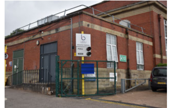
3.47 East Wing, substation building, east (R) and south (L) elevations
