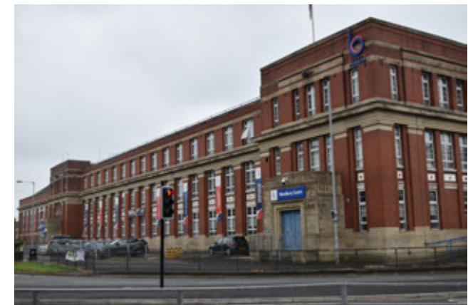
3.23 North pavilion (with entrance portico) and truncated east drive
