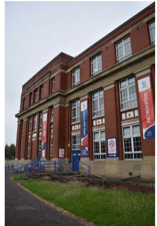
3.49 North elevation, projecting north pavilion
