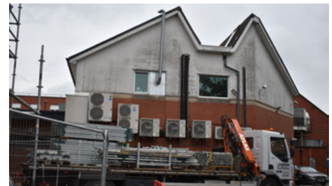
3.57 Modern rear range (Catering Wing), west elevation
