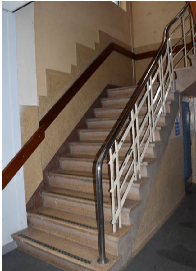
3.76 West exit stairs
