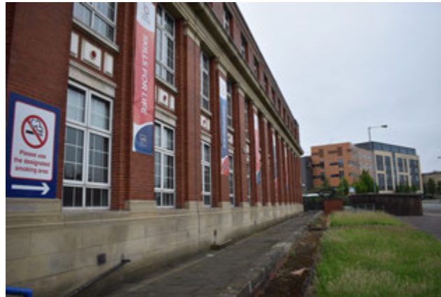
3.20 North elevation, former walled pathway
