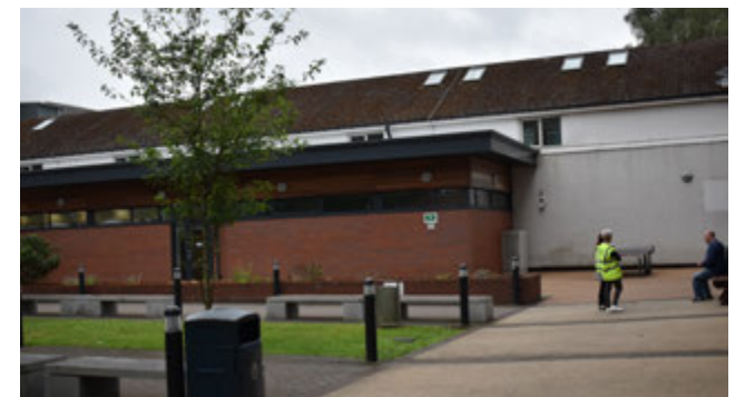
3.58 Modern rear ranges (Catering Wing), north elevations
