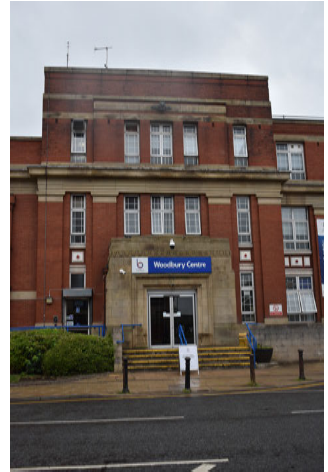
3.42 East Wing, east elevation, south entrance portico
