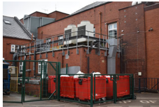
3.52 East Wing, rear (west), single-storey structure
