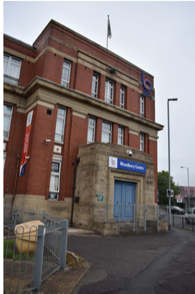
3.41 North Wing, east elevation, north pavilion and entrance portico
