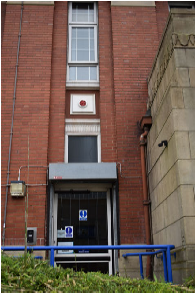
3.43 East Wing, east elevation, altered fenestration to the south of the south entrance portico to provide wheelchair access
