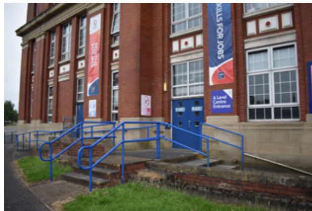
3.21 North elevation, inserted entrances with modern ramps, steps and railings, and truncated footpath and wall
