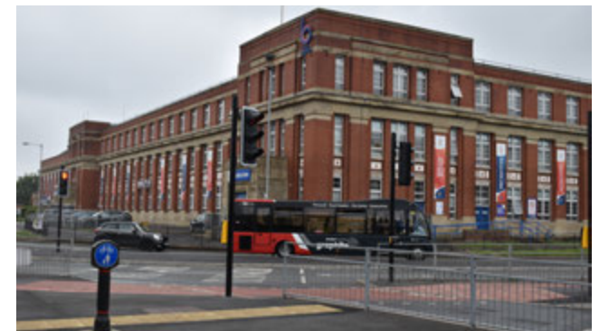
3.4 Complex crossings to the east and north, with a multiplicity of street furniture
