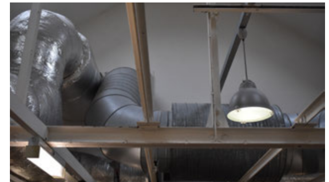
3.80 Former Gymnasium, ducting
