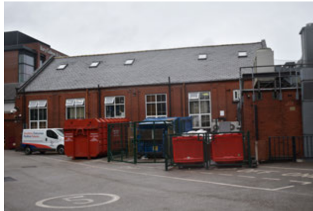
3.53 Former Gymnasium, south elevation
