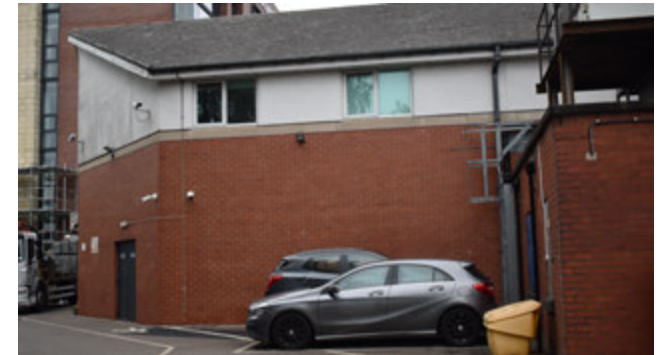
3.56 Modern rear range (Catering Wing), south and west elevations
