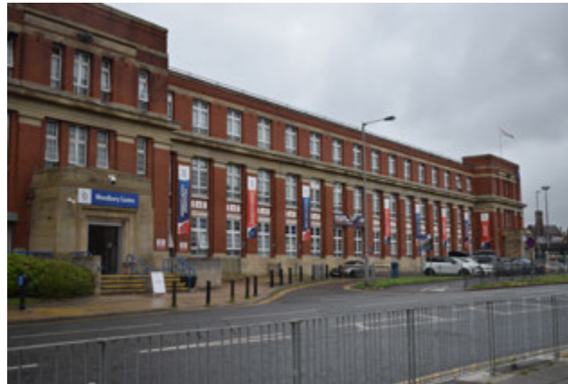
3.27 East car park
