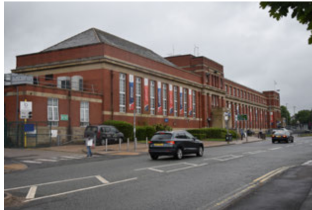
3.45 East Wing, east elevation (with North Wing, east elevation to the north)
