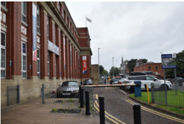
3.25 East car park and access road
