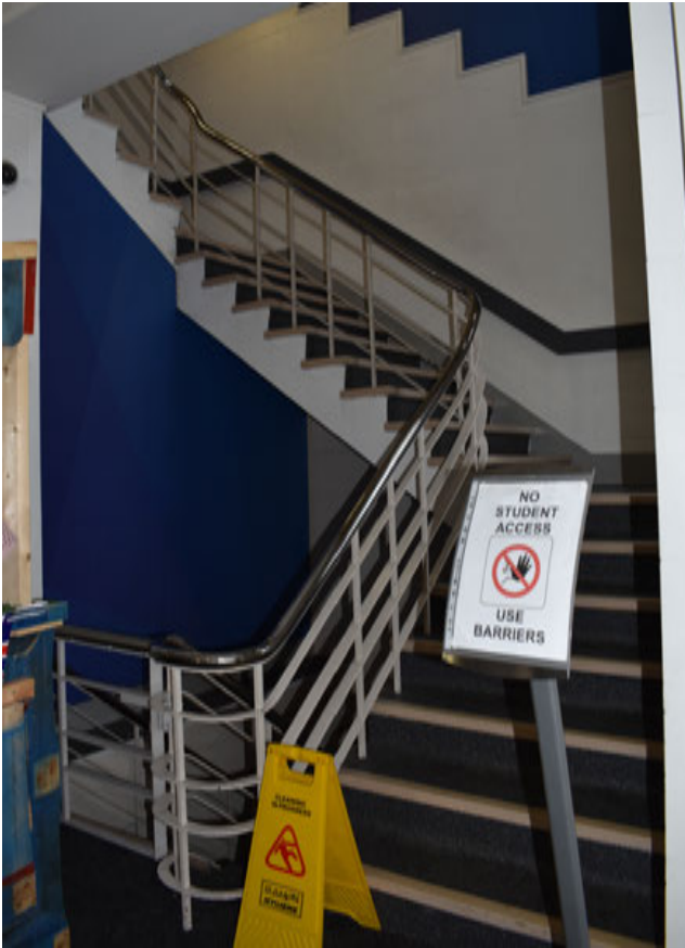
3.75 South entrance stairs
