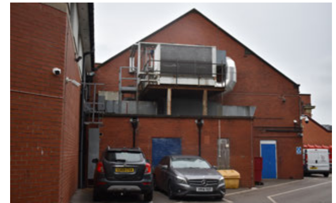
3.55 (Former) Gymnasium, west elevation
