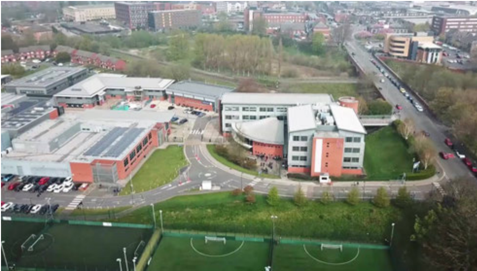
2.5 North (Woodbury) and south campuses, divided by Pyramid Park, 2019 (Bury College)
