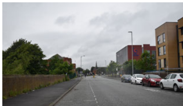
3.8 Market Street looking north, with contemporary college buildings to its east
