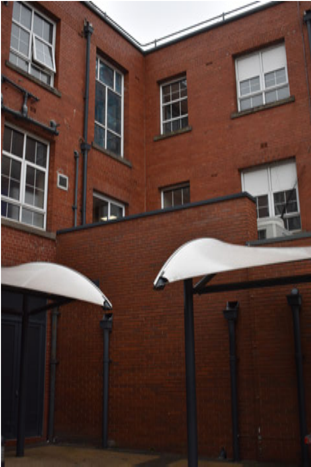
3.62 East Wing, west elevation, single-storey projection with plant (at juncture with North Wing)
