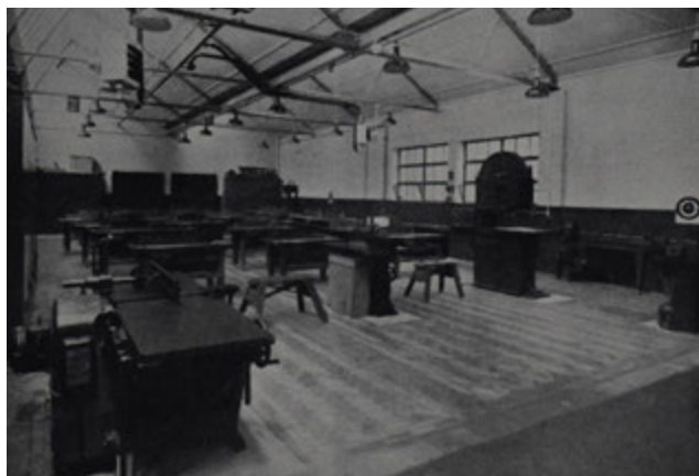
2.11 Carpentry and Joinery Workshop, 1947 (Bury Archives)
