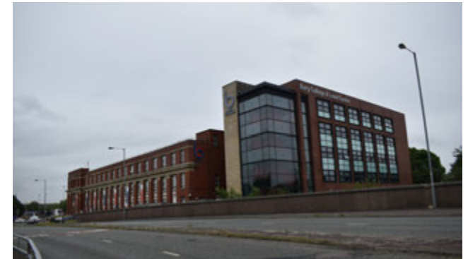
3.19 A Level Centre, west elevation
