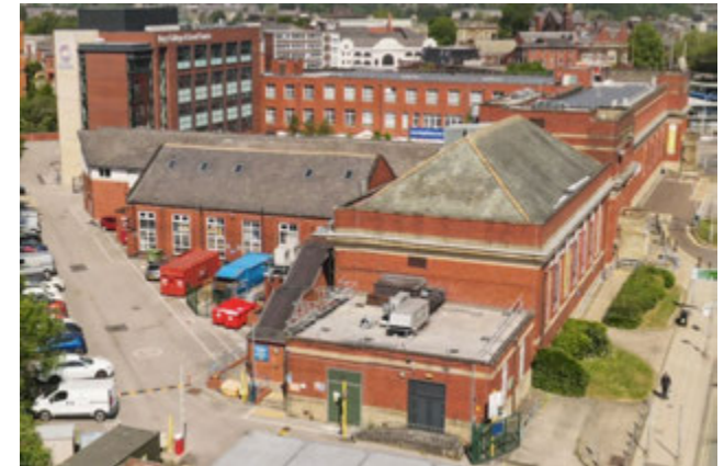
3.64 Woodbury Centre roofs, c.2021 (Bury College)
