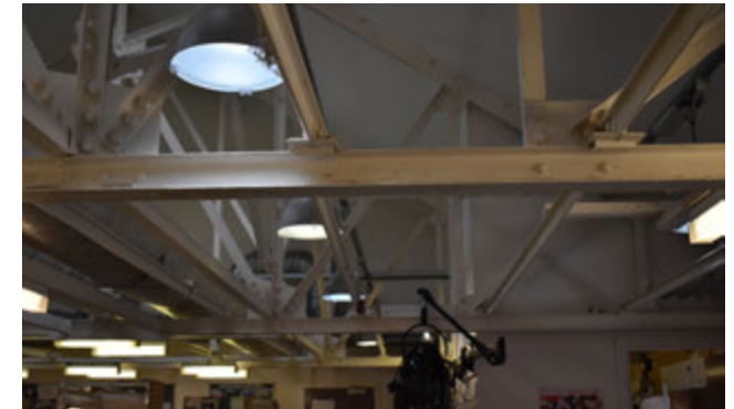
3.79 Former Gymnasium, exposed metal roof structure, with lighting and ducting attached
