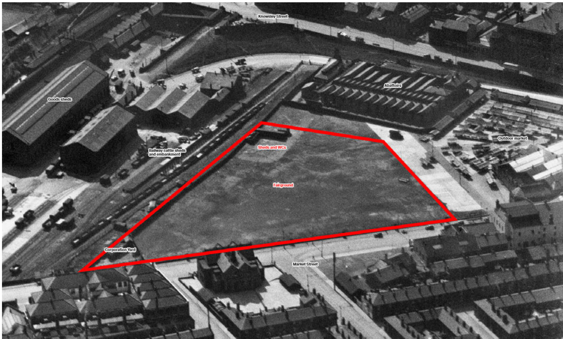
1.4 Future site of first college buildings (looking west), 1935 (Historic Scotland)
