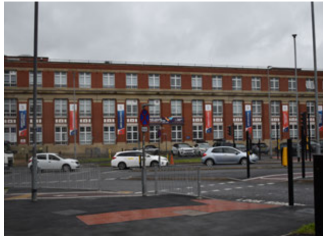
3.39 East Wing, east elevation, main range
