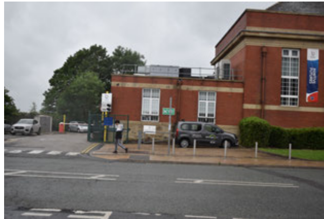
3.30 Service road entrance into the rear
