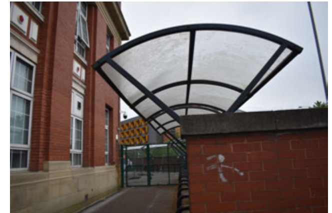
3.22 North elevation, cycle shelters and security gate
