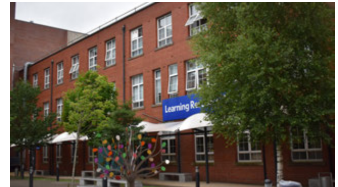
3.60 North Wing, south elevation, looking west
