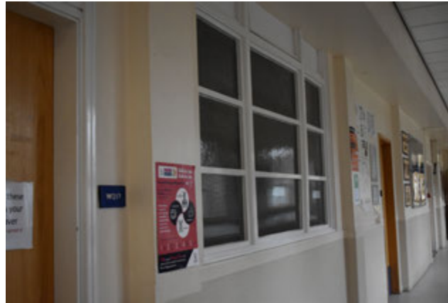
3.72 Room 212, Window to corridor
