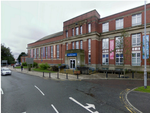
Low key, modest entrance, separate wheelchair access
