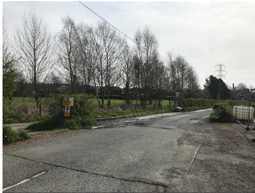
SOUTH EAST VIEW DOWN HOLLYMOUNT LANE
