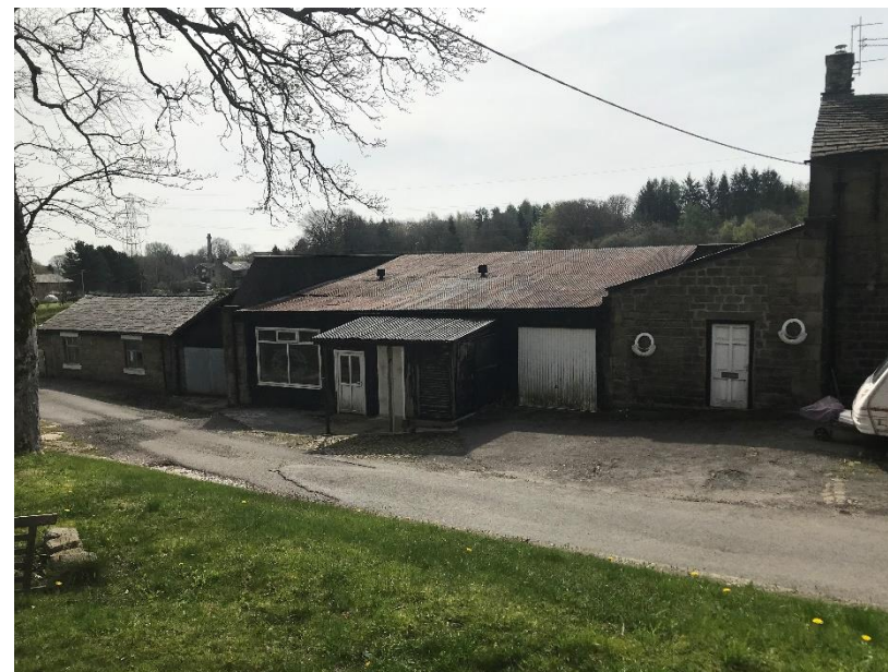
SOUTH VIEW OF BARN TO BE CONVERTED AND EXTENDED
