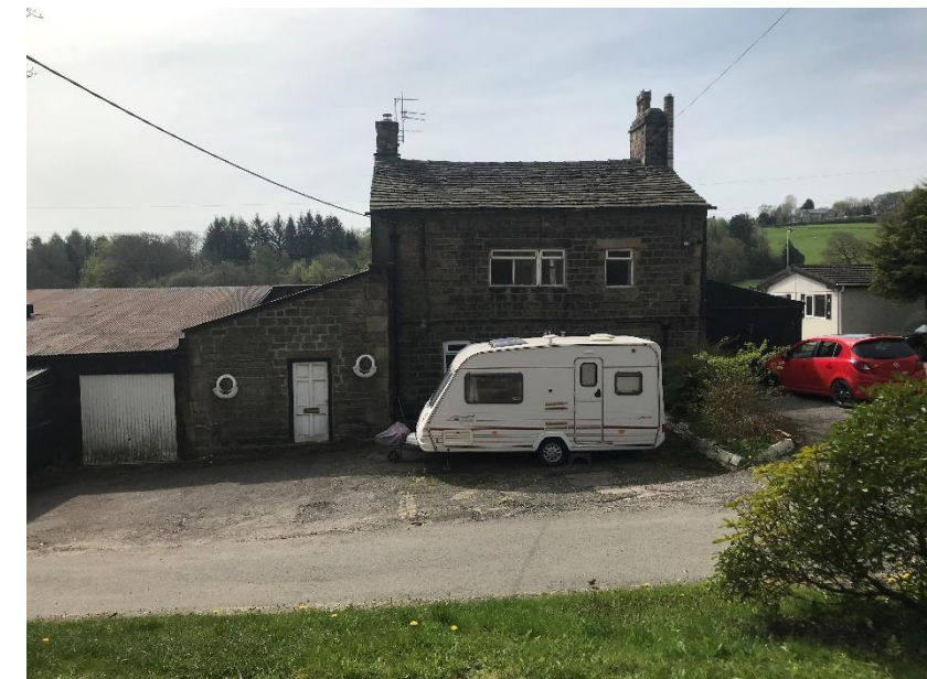
SOUTH VIEW OF FARMHOUSE TO BE EXTENDED
