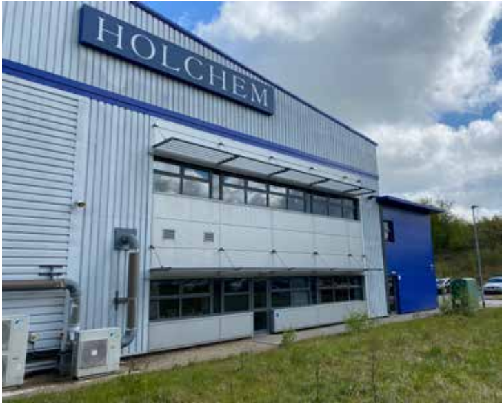
Existing windows on the building facade and external MEP
