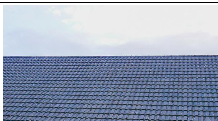
9. Rear roof in very good condition with no access opportunity for bats
