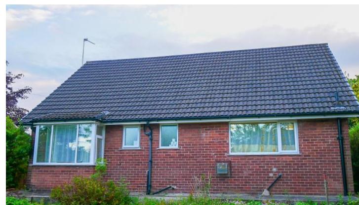
3. Rear elevation roof
