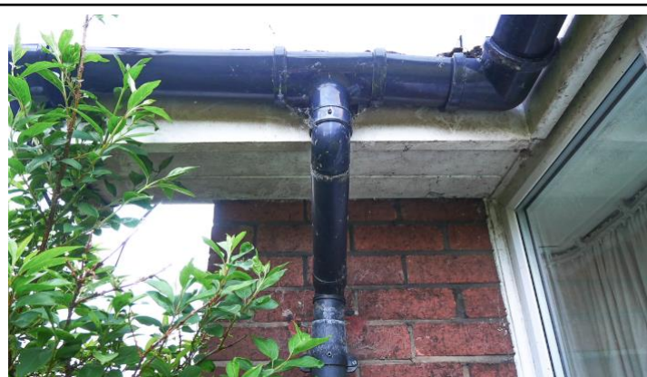
5. Gutters and drain pipes all in good order
