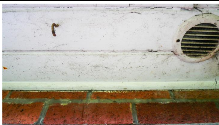
4. Ventilation grills in soffit boxes with no gaps or cracks preventing access by bats
