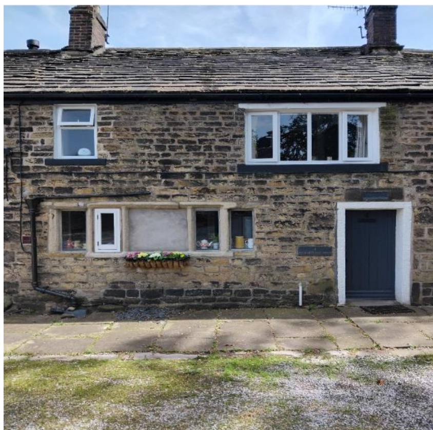
Front View of No 4 from the North
