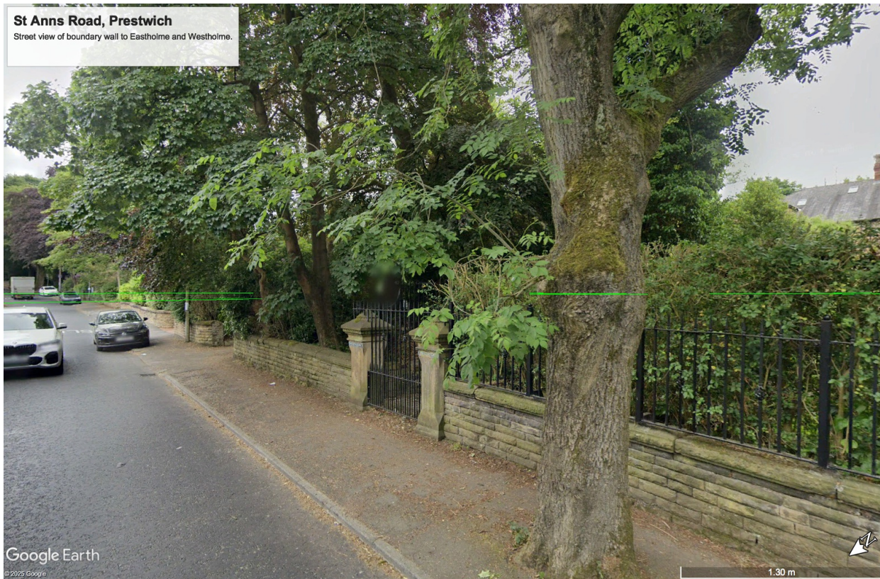
Google Earth image of the original wall
