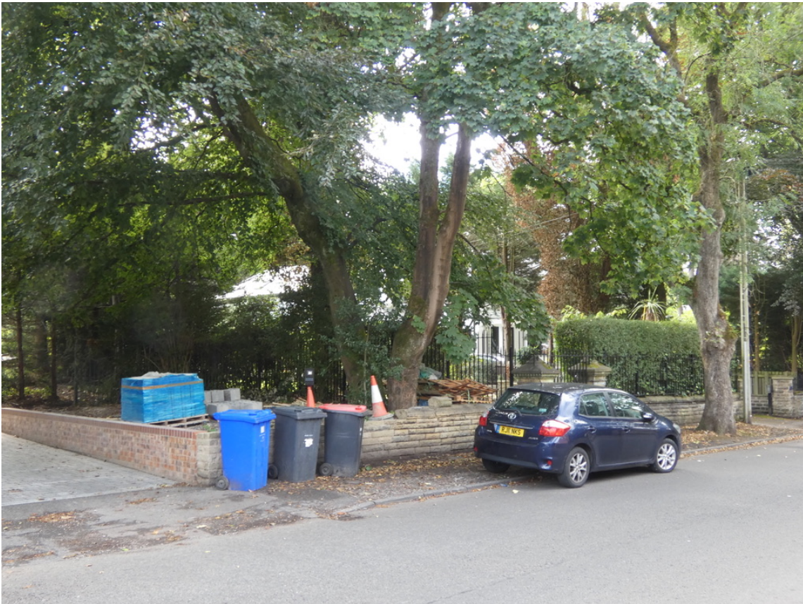
Current view of the boundary wall
