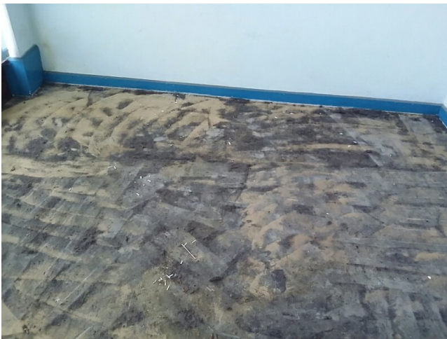
Sample No: 21/11/B/25/PK1 G.02 Office Floor Sheet vinyl flooring No Asbestos Detected
