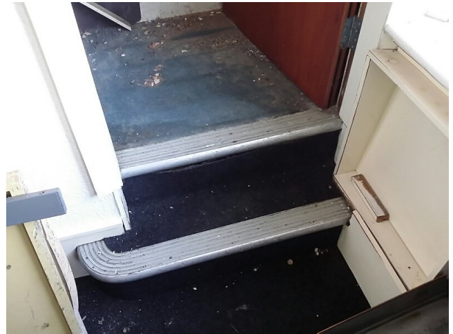
Sample No: 21/11/B/25/PK10 1.10 Stairwell Stairs Vinyl nosings No Asbestos Detected
