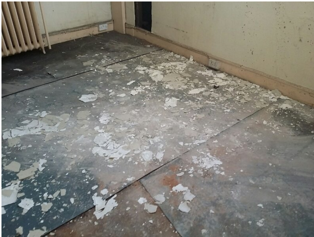
Sample No: Refer to Sample 21/11/B/25/PK5 2.12 Store Floor VFC No Asbestos Detected
