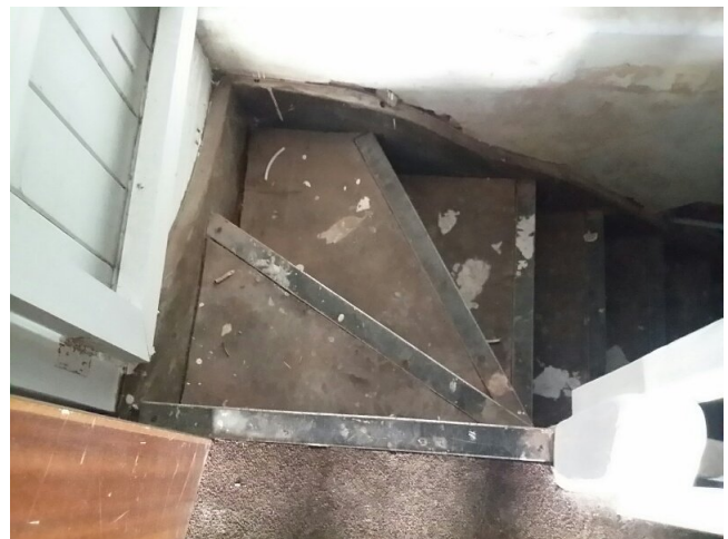
Sample No: 21/11/B/25/PK18 G.07 Basement stairwell Stairs Vinyl nosing No Asbestos Detected
