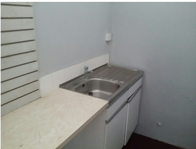
Sample No: 21/11/B/25/PK17 G.06 Shop unit Sink Bitumen pad No Asbestos Detected
