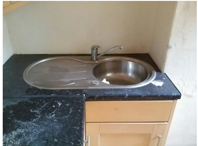
Sample No: 21/11/B/25/PK20 G.09 Kitchen area Sink Bitumen pad No Asbestos Detected
