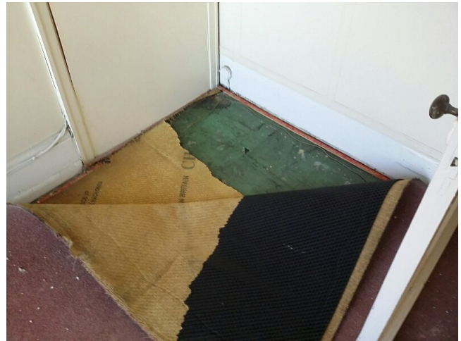
Sample No: 21/11/B/25/PK13 1.14 Office Floor Vinyl tiles below carpet containing: Chrysotile (In bitumen only)
