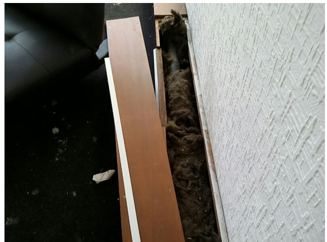
Sample No: 21/11/B/25/PK15 1.18 Office Pipe boxing Insulation to pipework No Asbestos Detected
