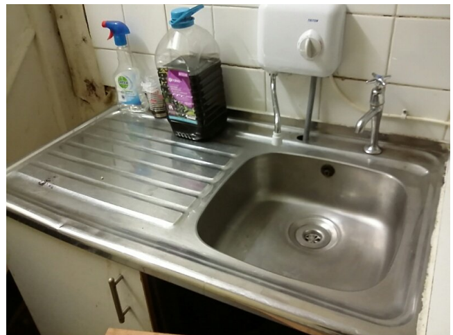
Sample No: 21/11/B/25/PK23 B.08 Store Sink Bitumen pad No Asbestos Detected
