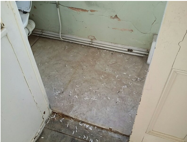
Sample No: 21/11/B/25/PK3 1.09 WC Floor WC No Asbestos Detected
