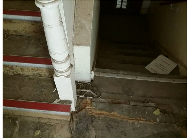
Sample No: 21/11/B/25/PK2 G.05 Stairwell Stairs Vinyl nosings No Asbestos Detected
