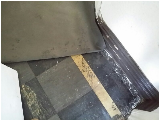
Sample No: Refer to Sample 21/11/B/25/PK12 1.13 Circulation Floor below carpet Vinyl floor tiles No Asbestos Detected
