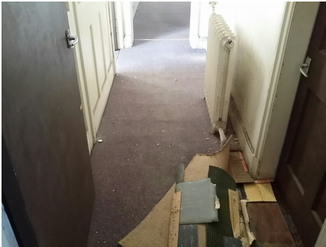
Sample No: 21/11/B/25/PK8 2.08 Corridor Floor Core sample (various floor coverings) No Asbestos Detected
