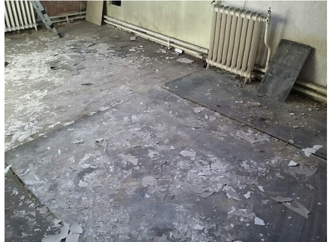
Sample No: 21/11/B/25/PK5 2.02 Store Floor VFC No Asbestos Detected
