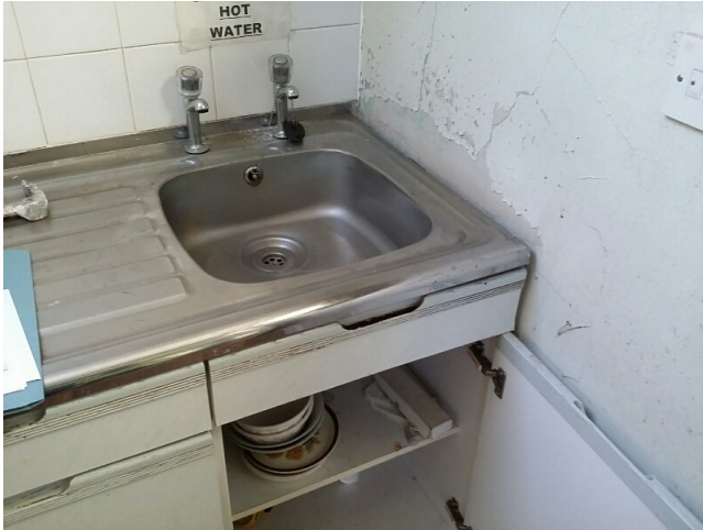
Sample No: 21/11/B/25/PK4 2.01 Kitchen Sink Bitumen pad No Asbestos Detected
