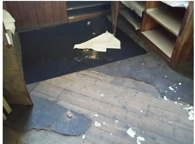
Sample No: Refer to Sample 21/11/B/25/PK5 2.14 Store Floor VFC No Asbestos Detected
