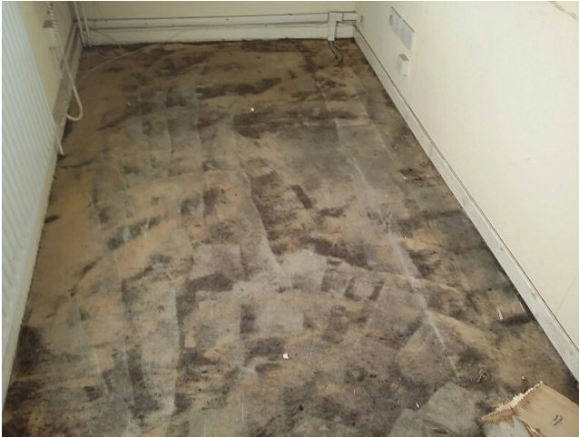
Sample No: Refer to Sample 21/11/B/25/PK1 G.04 WC Floor Sheet vinyl flooring No Asbestos Detected
