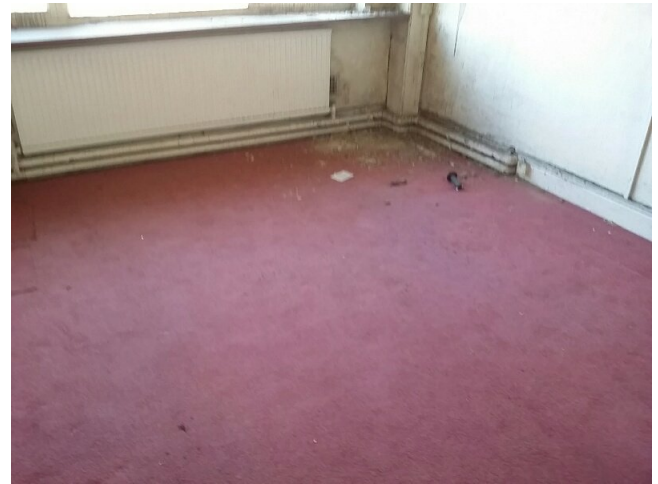
Sample No: 21/11/B/25/PK9 2.09 Office Floor VFC below carpet No Asbestos Detected
