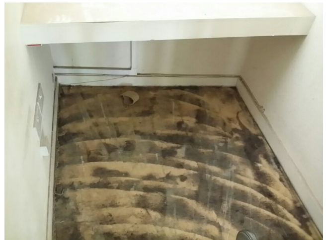
Sample No: Refer to Sample 21/11/B/25/PK1 G.03 Office Floor Sheet vinyl flooring No Asbestos Detected
