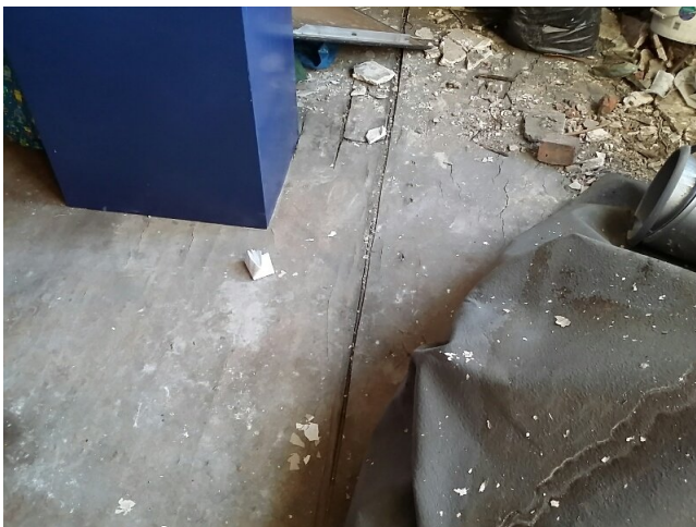
Sample No: 21/11/B/25/PK14 1.16 Office Floor VFC No Asbestos Detected
