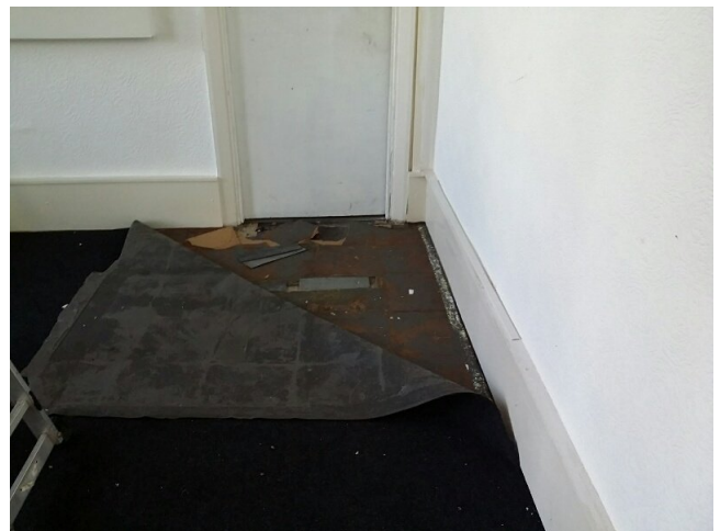
Sample No: 21/11/B/25/PK12 1.11 Store Floor below carpet Vinyl floor tiles No Asbestos Detected
