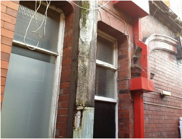
Sample No: 21/11/B/25/PK16 External Court yard Insulation to pipe in boxing No Asbestos Detected
