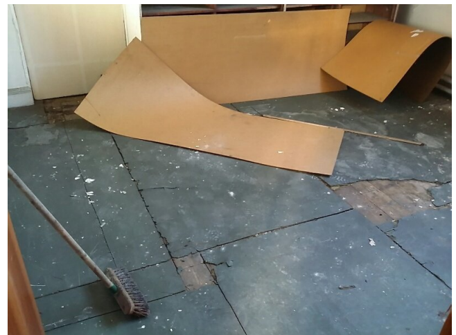
Sample No: Refer to Sample 21/11/B/25/PK5 2.11 Store Floor VFC No Asbestos Detected
