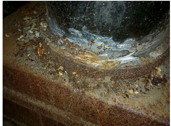
Sample No: 22/3/B/8/IL1. B.01 Basement Area 1 - Plant Corridor - Gas Boiler. Woven gasket & mastic seal to gas boiler / metal flue joint. No Asbestos Detected
