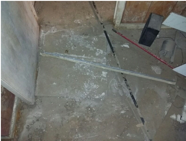
Sample No: 22/3/B/9/IL17. B.02 Basement Area 2 - Office – Floor. Vinyl floor covering & paper backing. No Asbestos Detected.
