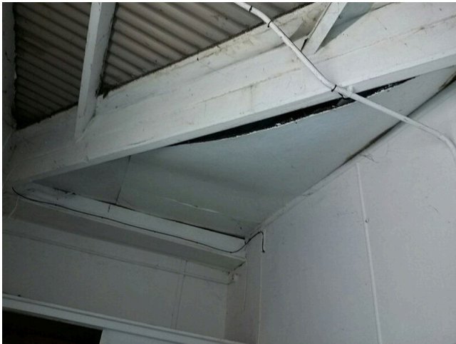
Refer to Sample 22/3/B/9/IL21. G.03 Corridor – Ceiling. Fibreboard roof lining boards. No Asbestos Detected.
