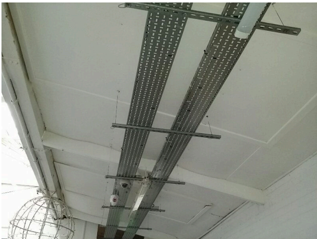
Refer to Sample 22/3/B/9/IL21. G.02 Market Hall Circulation Area – Ceiling. Fibreboard roof lining boards. No Asbestos Detected.
