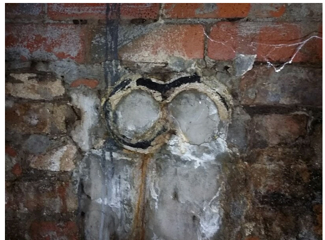
Sample No: 22/3/B/9/IL20. B.02 Basement Area 2 - Basement Circulation - Wall penetration. Thermoplastic & Composite linings. No Asbestos Detected.
