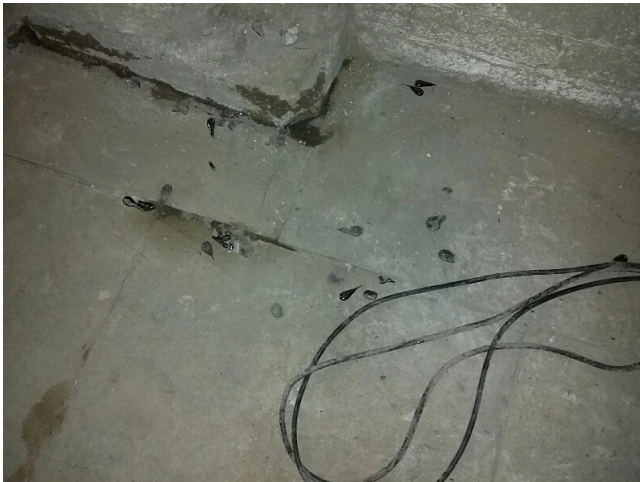
Sample No: 22/3/B/9/IL16. B.01 Basement Area 1 - Basement Shelter - Floor & Surfaces. Residual bitumen & debris. No Asbestos Detected.
