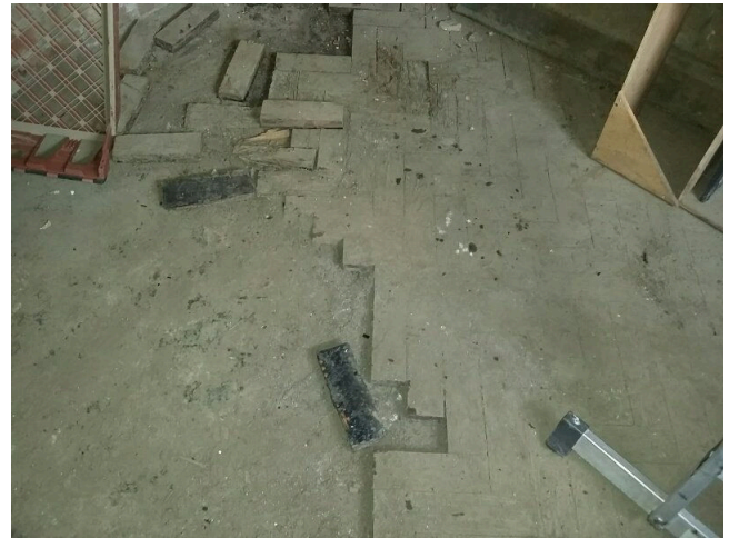
Sample No: 22/3/B/8/IL9. B.01 Basement Area 1 - Store – Floor. Bitumen adhesive to parquet flooring. No Asbestos Detected.
