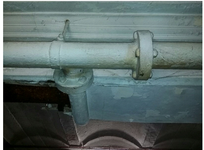
Refer to Sample 22/3/B/8/IL11. B.01 Basement Area 1 - Large Store – Pipework. Mastic sealant to pipework flanges. No Asbestos Detected.
