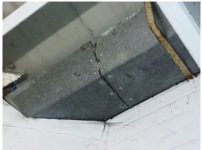
Sample No: 22/3/B/9/IL23. G.03 Corridor - Rainwater gutter. Mastic seal to joints. No Asbestos Detected.
