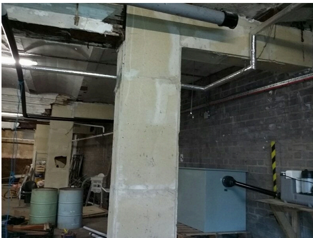
Sample No: 22/3/B/8/IL10. B.01 Basement Area 1 - Large Store - Structural steelwork. Insulating board cladding to columns & beams (Vicucad). No Asbestos Detected.
