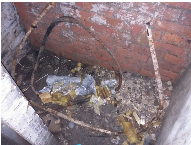
Sample No: 22/3/B/9/IL19. B.02 Basement Area 2 - Basement Store - Electric Cable. Woven insulation to redundant cable. No Asbestos Detected.
