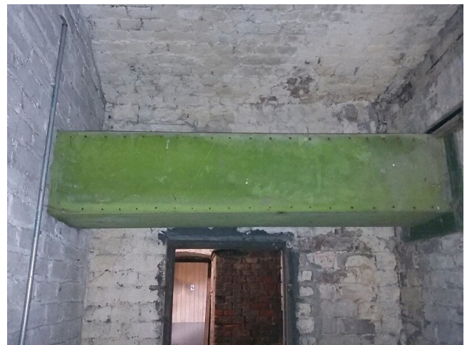
Sample No: 22/3/B/9/IL15. B.01 Basement Area 1 - Basement Shelter – Ducting. Organic ducting panels. No Asbestos Detected.
