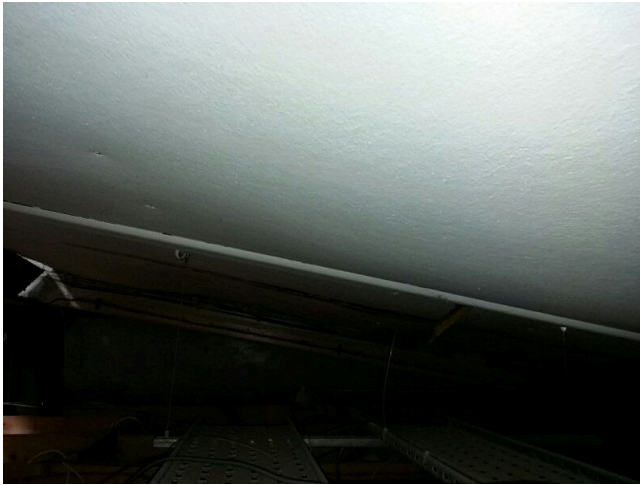
Sample No: 22/3/B/9/IL21. G.01 Entrance Lobby - Ceiling void. Fibreboard roof lining boards. No Asbestos Detected.
