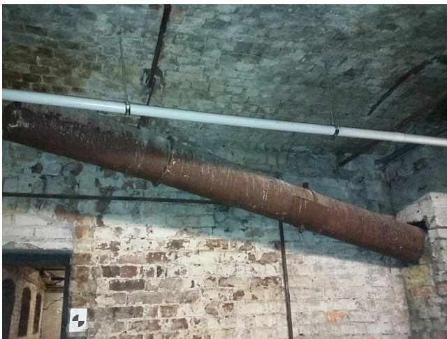
Sample No: 22/3/B/9/IL14. B.01 Basement Area 1 - Old Boiler Room - Redundant metal flue pipe. Residuals to flue pipe. No Asbestos Detected.
