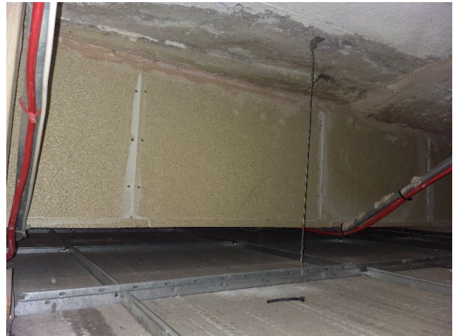
Sample No: Refer to Sample 22/3/B/22/PK9 B.03 Welfare / kitchen Ceiling void Insulation board cladding to beams No Asbestos Detected
