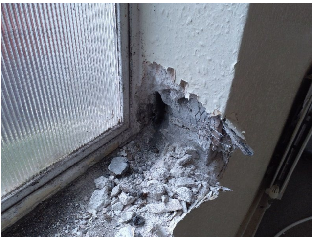
Sample No: 22/4/B/4/PK17 1.02 Corridor External walls Bitumen vapour barrier No Asbestos Detected
