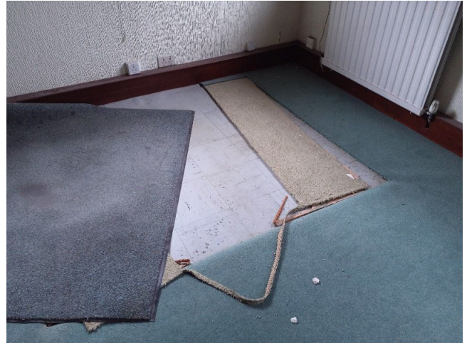
Sample No: Refer to Sample 22/4/B/4/PK16 1.04 Office Floor VFTs below carpet No Asbestos Detected
