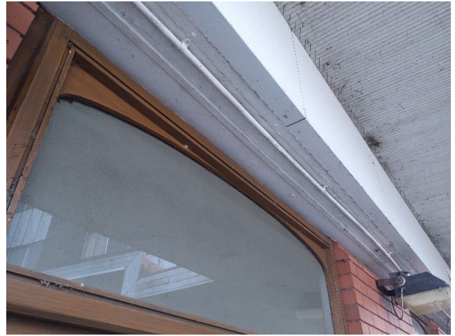
Sample No: 22/3/B/22/PK11 External Soffit above windows Soffit panels No Asbestos Detected
