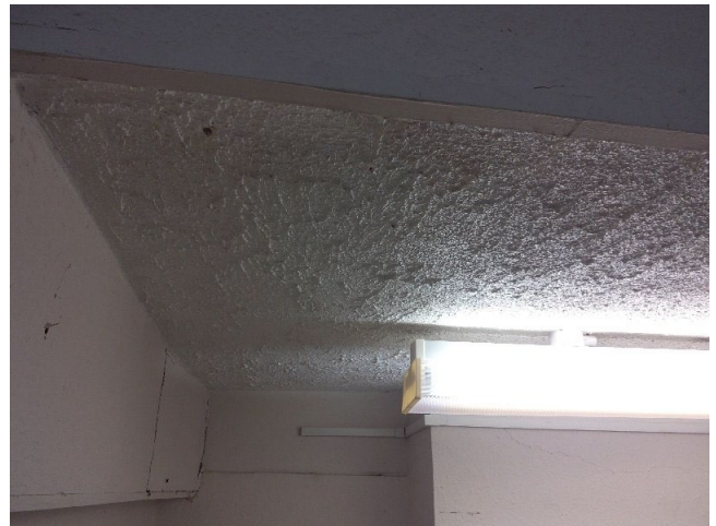
Sample No: 22/3/B/21/PK1 B.01 Stairwell Ceiling Textured coating No Asbestos Detected
