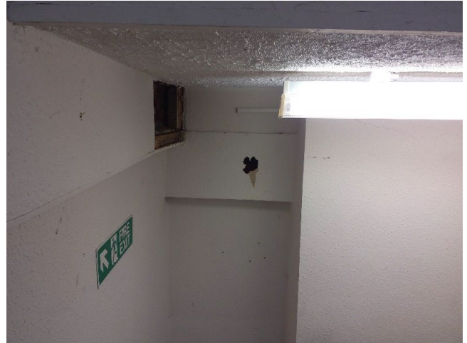
Sample No: 22/3/B/22/PK9 B.01 Stairwell Wall Insulation board cladding No Asbestos Detected
