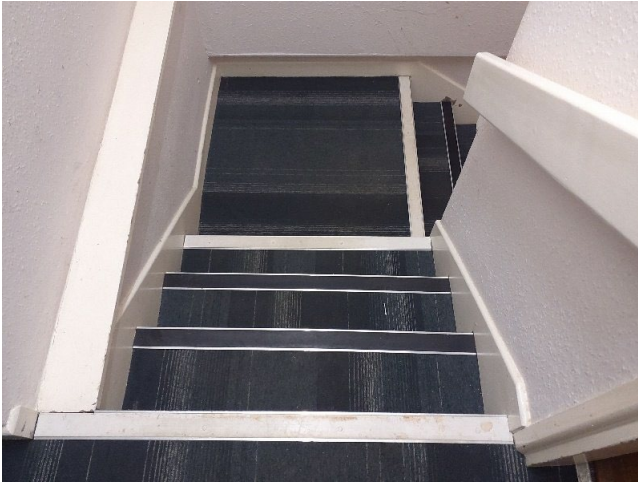
Sample No: 22/3/B/22/PK8 B.01 Stairwell Stairs Vinyl stair nosings No Asbestos Detected
