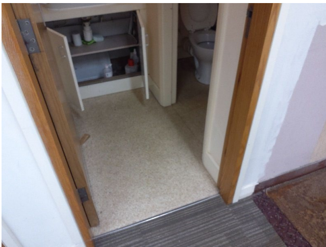
Sample No: Refer to Sample 22/3/B/21/PK7 G.09 Female WC Floor VFC No Asbestos Detected
