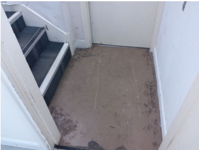
Sample No: 22/3/B/21/PK2 B.02 Circulation Floor VFC No Asbestos Detected
