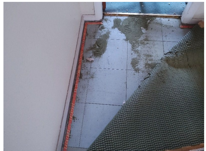
Sample No: Refer to Sample 22/4/B/4/PK16 1.02 Corridor Floor VFTs below carpet No Asbestos Detected
