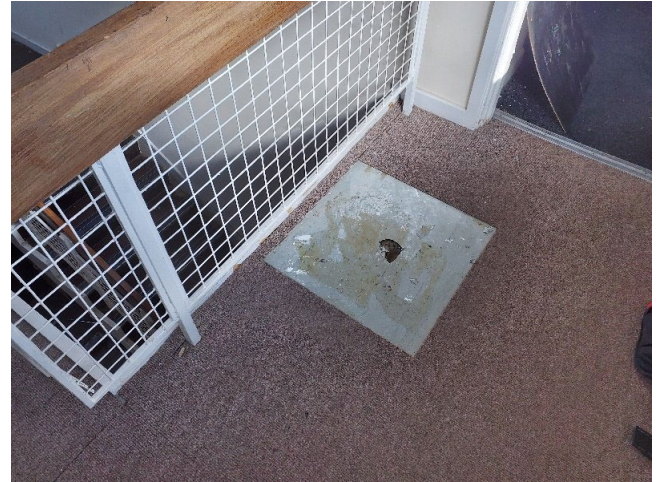
Sample No: 22/3/B/22/PK15 1.01 Stairwell lobby Floor VFC No Asbestos Detected
