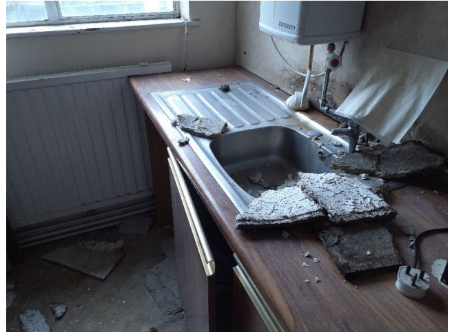
Sample No: 22/4/B/4/PK18 1.08 Kitchen Sink Bitumen pad No Asbestos Detected
