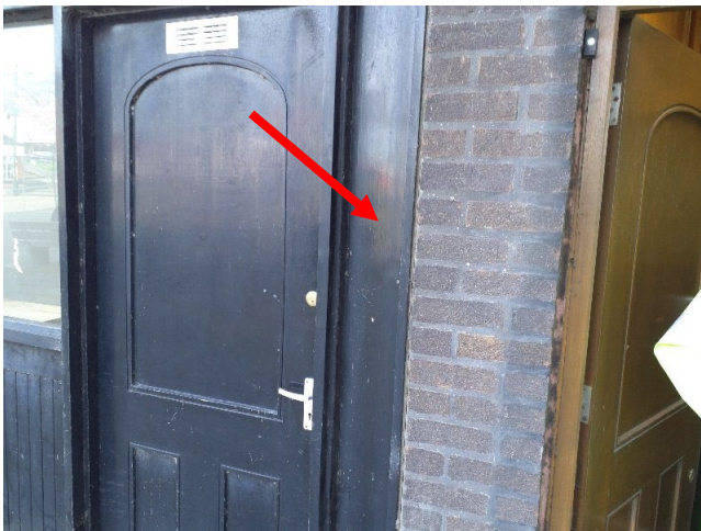
Sample No: 22/3/B/22/PK12 External RHS of door Fascia panel No Asbestos Detected
