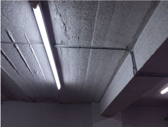
Sample No: 22/3/B/21/PK5 B.08 Store Ceiling Textured coating No Asbestos Detected
