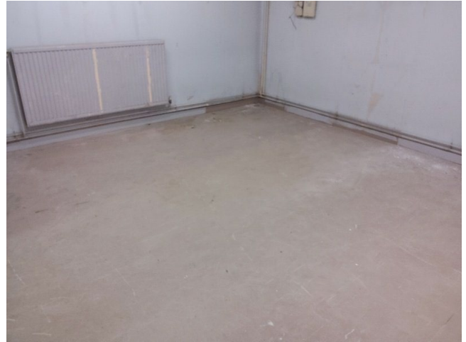
Sample No: Refer to Sample 22/3/B/21/PK2 B.08 Store Floor VFC No Asbestos Detected
