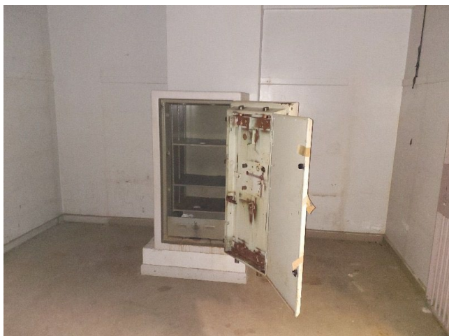
Safe in basement strong room (may have ACMs internally)
