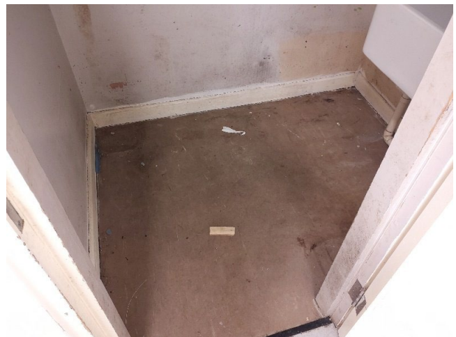
Sample No: Refer to Sample 22/3/B/21/PK2 B.05 Store Floor VFC No Asbestos Detected
