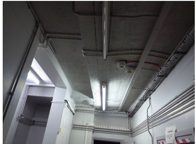
Sample No: Refer to Sample 22/3/B/21/PK1 B.06 Circulation Ceiling Textured coating No Asbestos Detected
