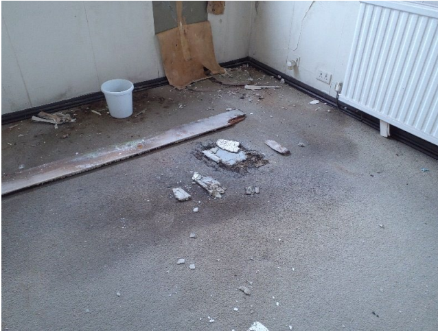
Sample No: Refer to Sample 22/4/B/4/PK16 1.07 Office Floor VFTs below carpet No Asbestos Detected
