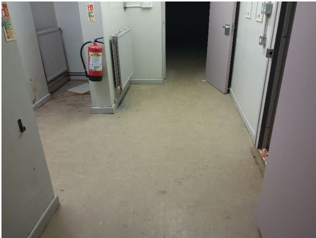
Sample No: Refer to Sample 22/3/B/21/PK2 B.06 Circulation Floor VFC No Asbestos Detected
