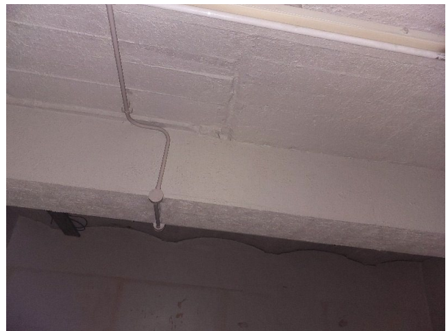
Sample No: Refer to Sample 22/3/B/21/PK1 B.07 Strong room Ceiling Textured coating No Asbestos Detected
