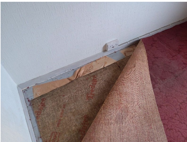
Sample No: Refer to Sample 22/4/B/4/PK16 1.05 Office Floor VFTs below carpet No Asbestos Detected
