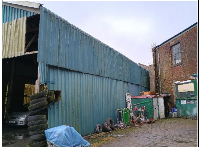
Photo 2: Eastern elevation of Building 1.
