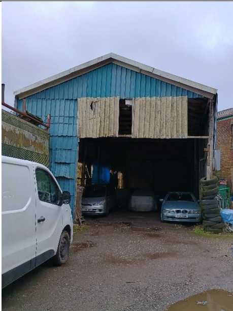
Photo 1: (28.01.25) Southern elevation of Building 1.
