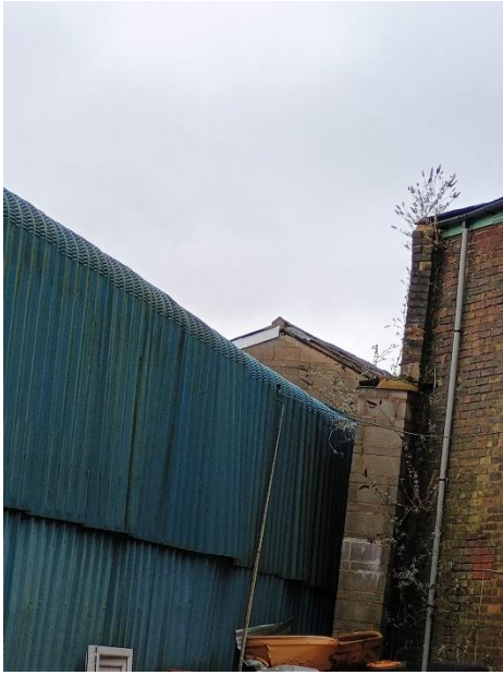
Photo 5: North-eastern corner of Building 1.
