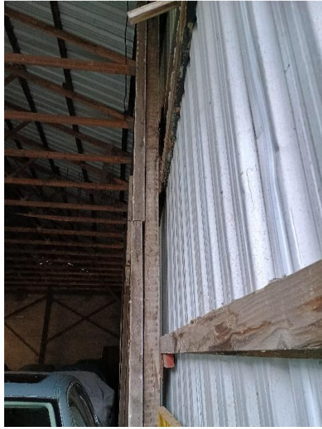
Photo 6: Wooden posts internally.
