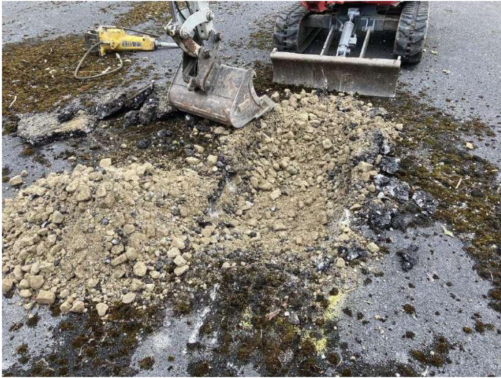
Plate 11 – TP4 gl to approximately 0.2mbgl with arisings
