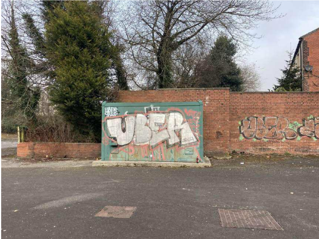
Plate 5 – Container in the south east corner of site. Note Services
