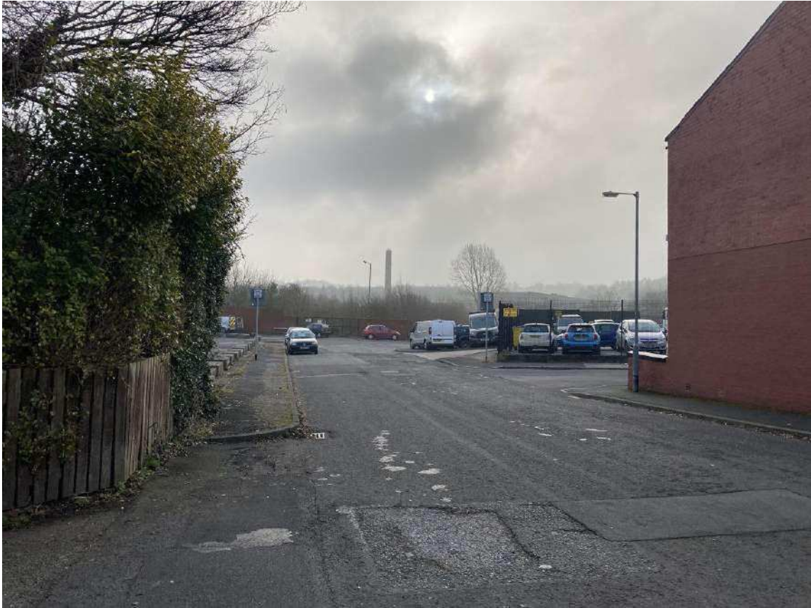
Plate 19 – Radcliffe street looking south
