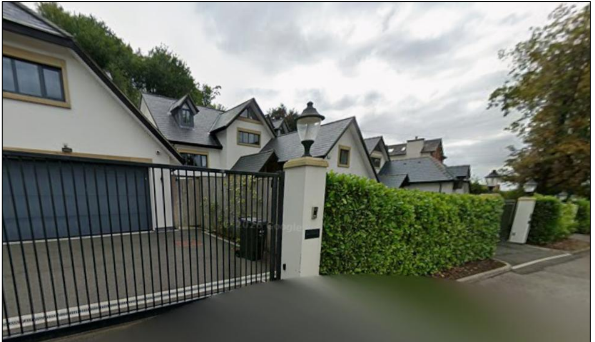
Figure 2: View towards the front elevation of the application property
