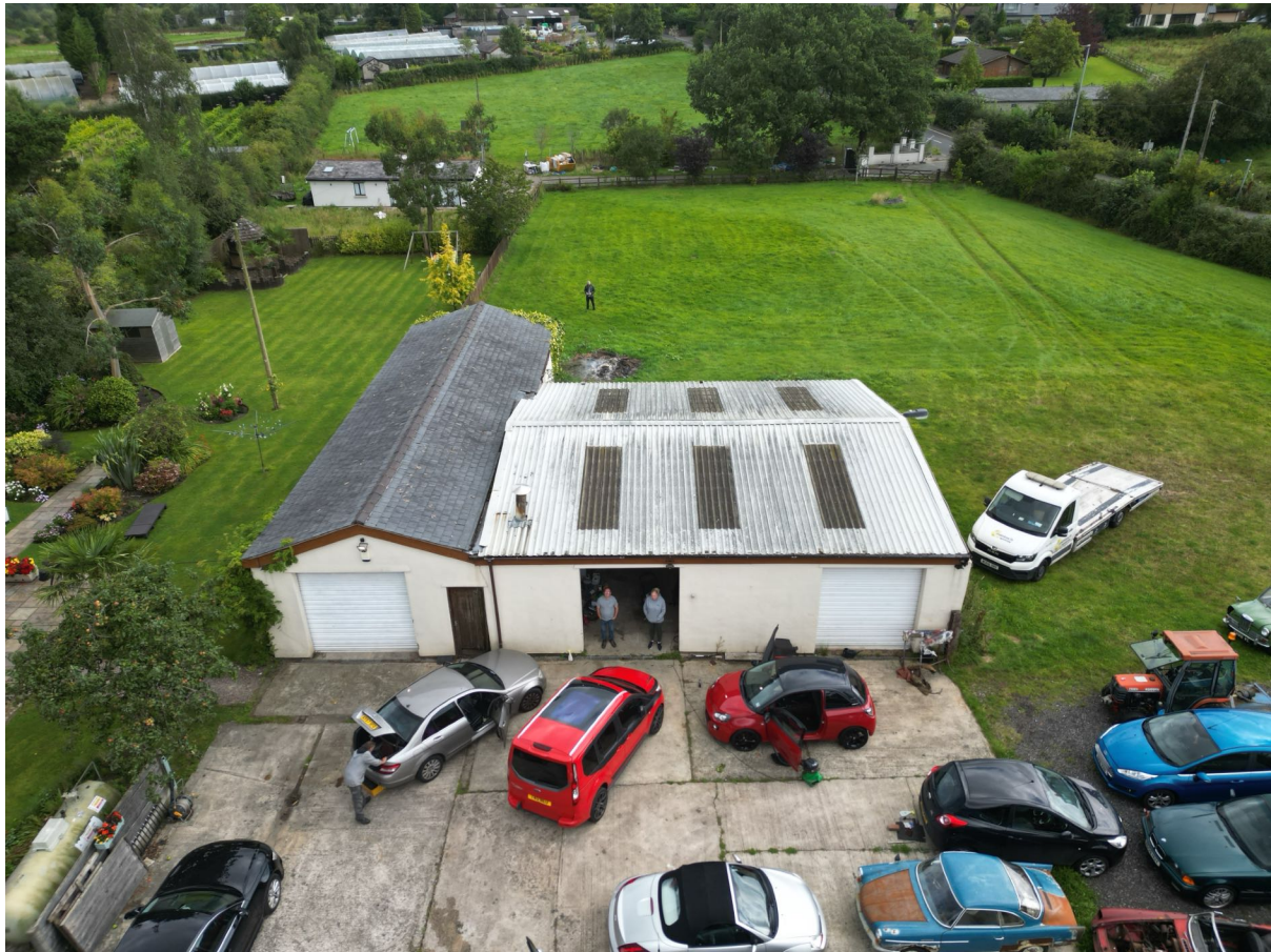
3.1a – The front of the garage.
