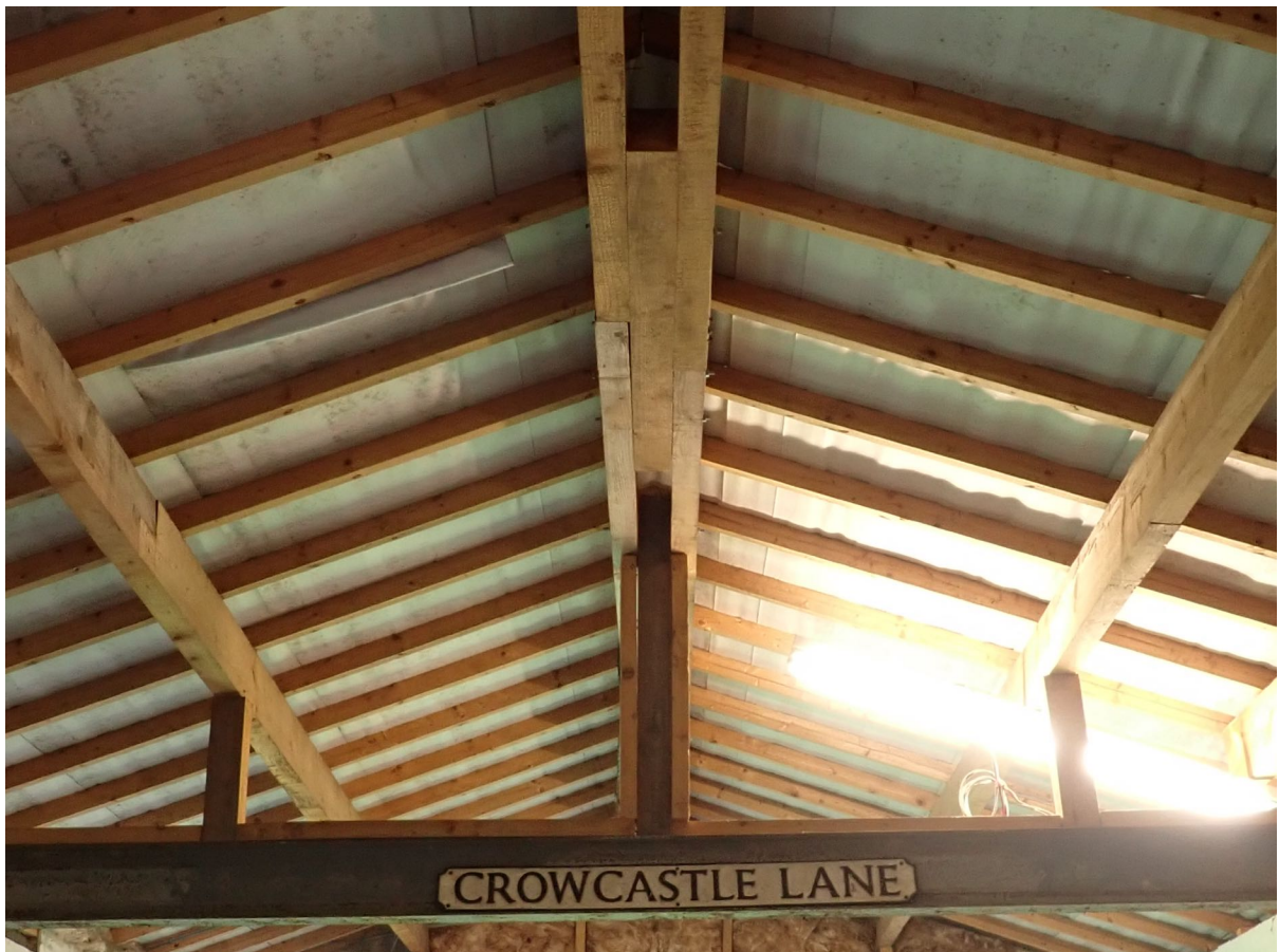
6 – The eastern section of the roof is lined with a modern breathable membrane.
