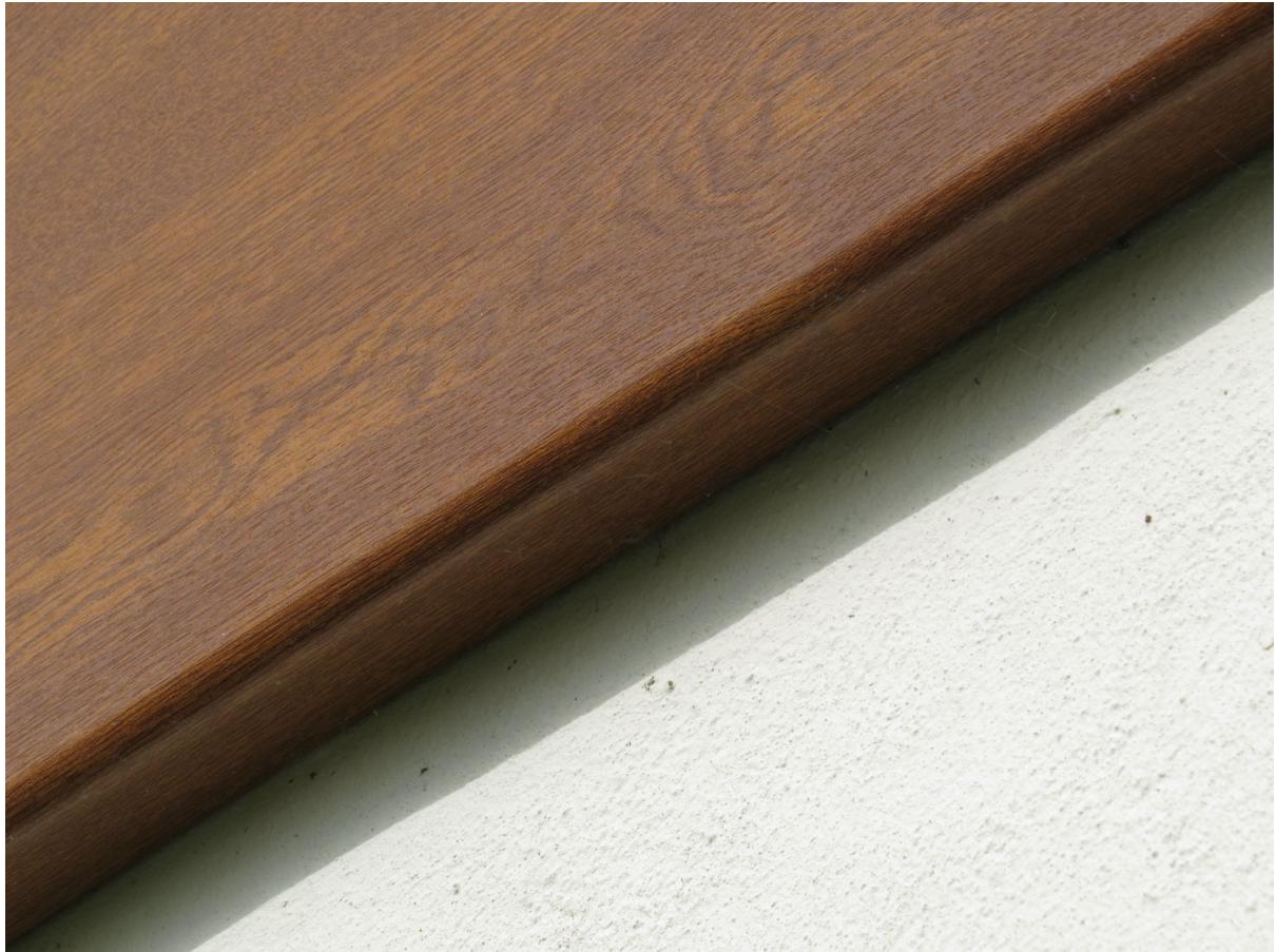
5 – UPVC fascia are tightly fitted with no suitable gaps.
