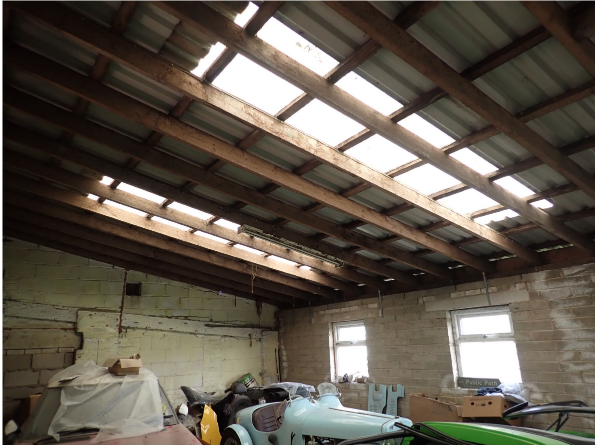
3.2a – Inside the garage.
