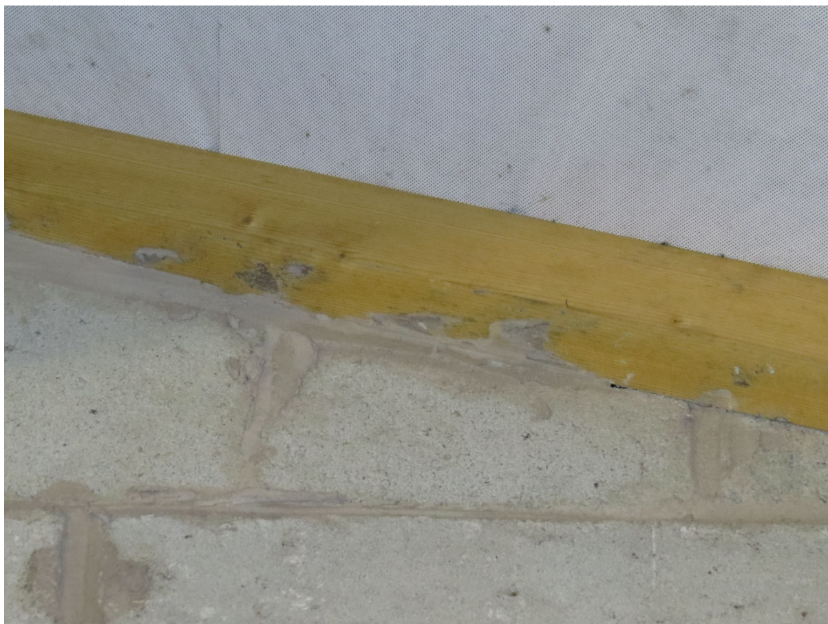
8 – Roof timbers are sealed against concrete block walls with no gaps.
