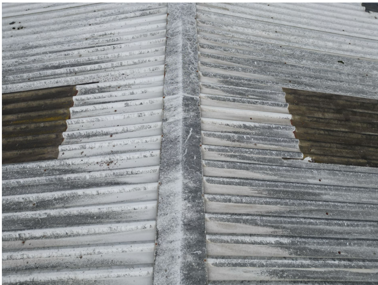
4 – Corrugated roof panels are fitted tightly with no gaps between panels.
