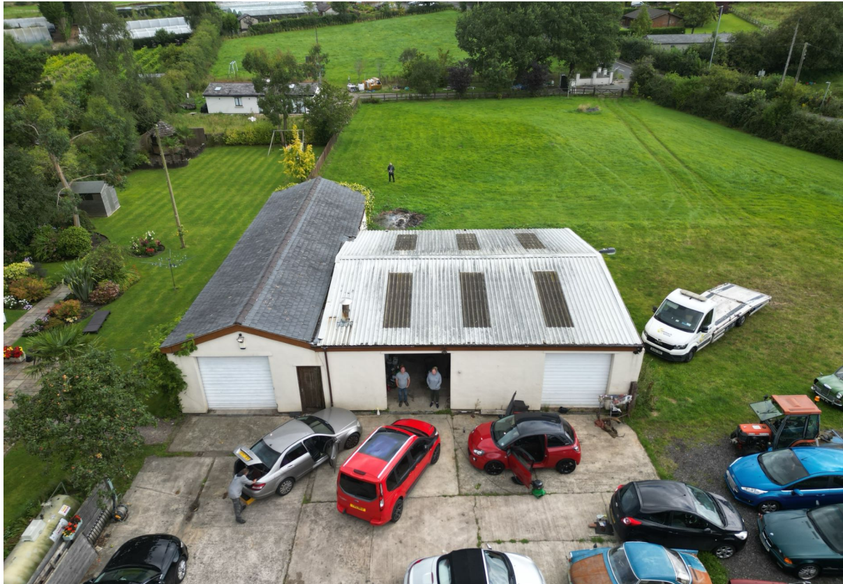
1 – The south side of the garage.
