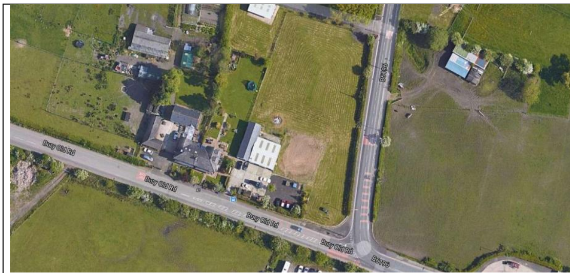
Figure 7 Above: Aerial photograph of site looking north eastwards across Bury Old Road and up Arthur Lane from south. The centre of the site is the brown square area (former menage area). The concrete hardstanding and hardcore parking areas are to the south and south-east of the former stables block
