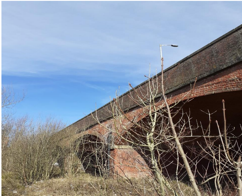
Figure 5: Market Street Arches
