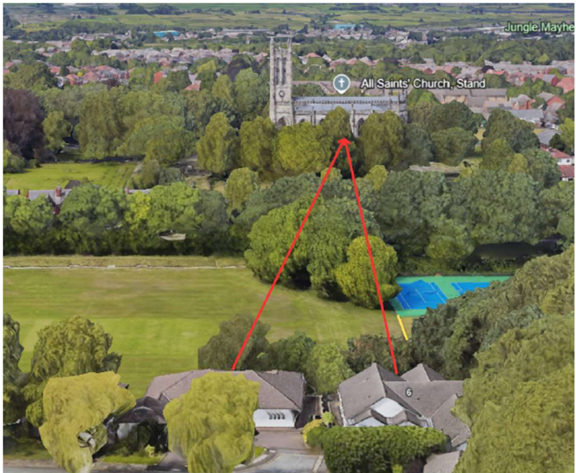
Figure 13 – View of All Saints Stand from Parklands No. 6, 7 & 8 not interrupted by planned site (yellow)
