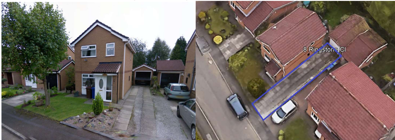
Figure 5 – Existing driveway/parking area
