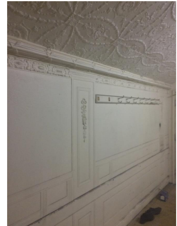
The decorative plasterwork on the walls and ceiling of the undeveloped space.
