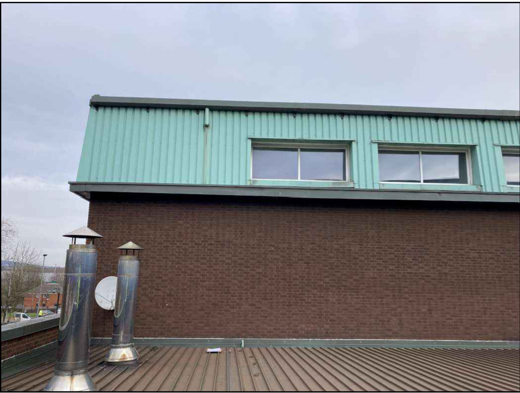
Photograph of Existing South Elevation
