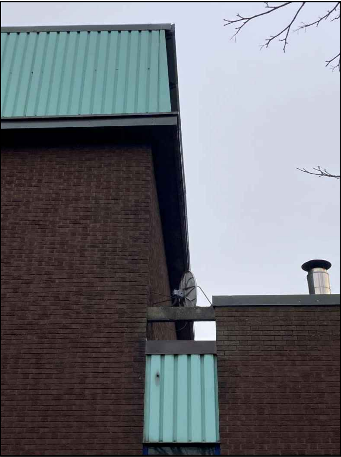
Photograph of Existing West Elevation
