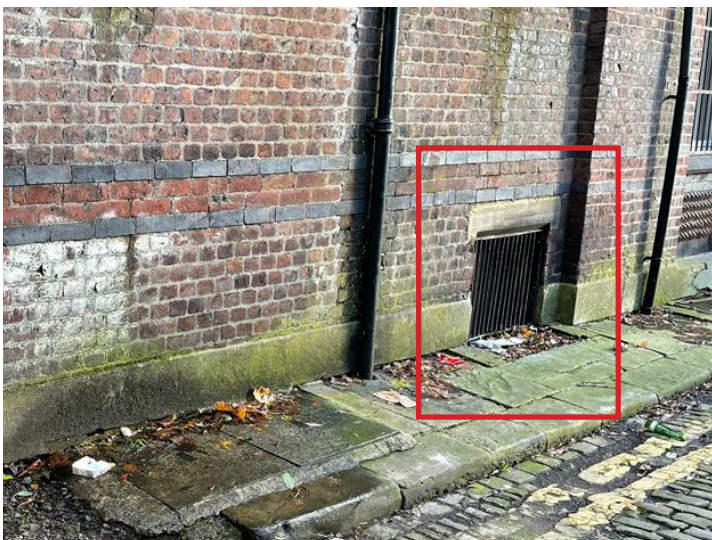
Existing basement windows that are to be reinstated.
