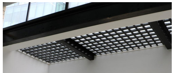
Examples of Cast Iron pavement lights
