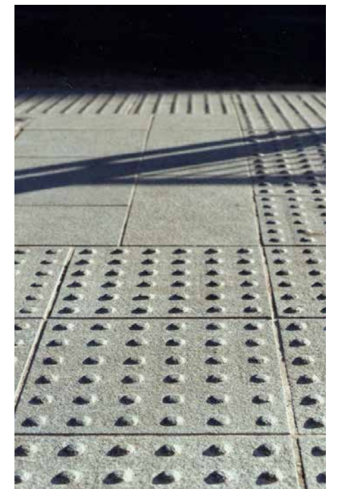
Granite Tactile Paving Flamed finish Colour: Tagenta B
