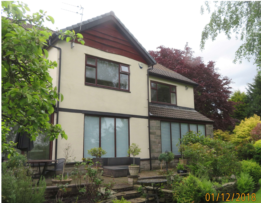
2. View of existing house from the garden
