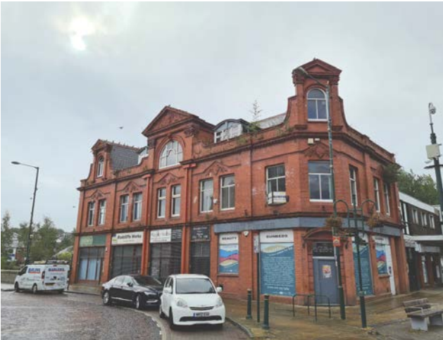
8 View of Radcliffe Market Chambers main elevation
