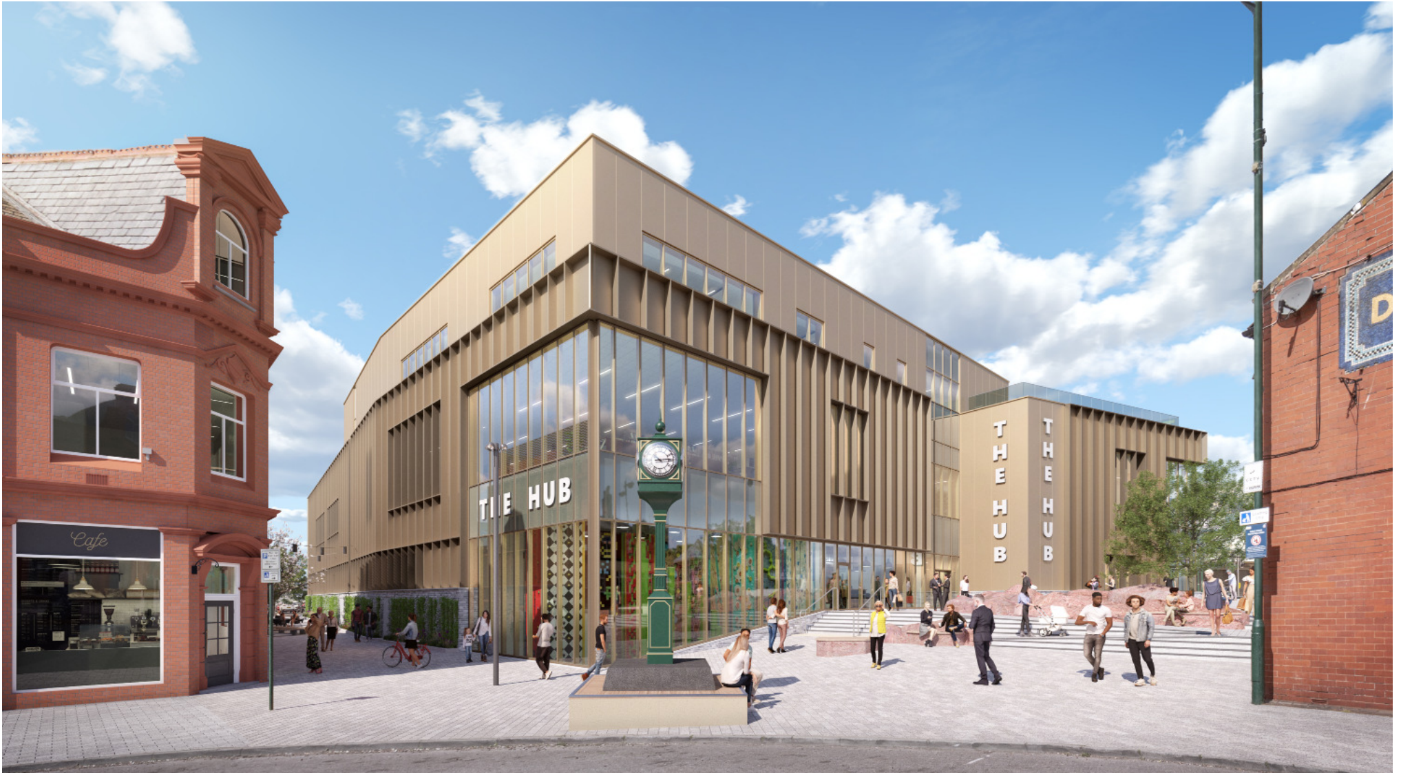
View of Civic Hub from corner of Blackburn Street and Church Street
