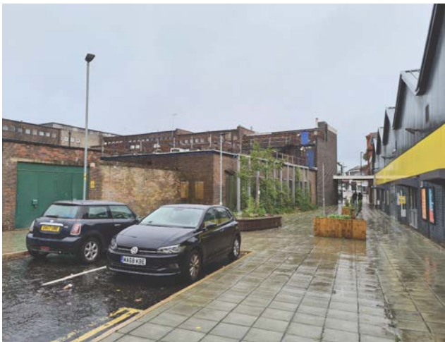
5 View north-east along main elevation of Radcliffe Market
