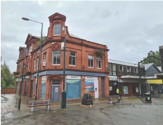
7 View of Radcliffe Market Chambers and link block site
