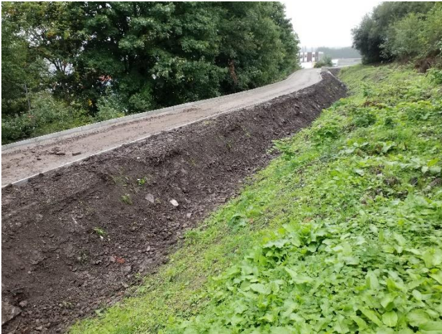
Figure 4.13: Bealey's Goit at northern extent of Scheme footprint
