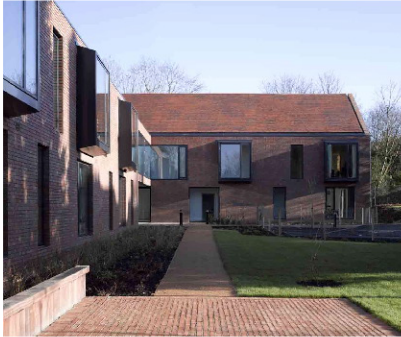
BOX BAY WINDOWS
