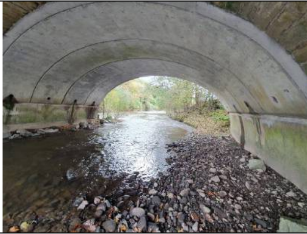
Photograph 7: Under the bridge north of survey Patch 5 of the River Irwell, October 2019.
