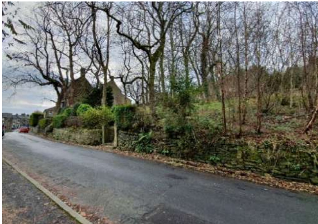
November 2019- view of tanners St looking South West towards 12 & 12a and pedestrian access steps
