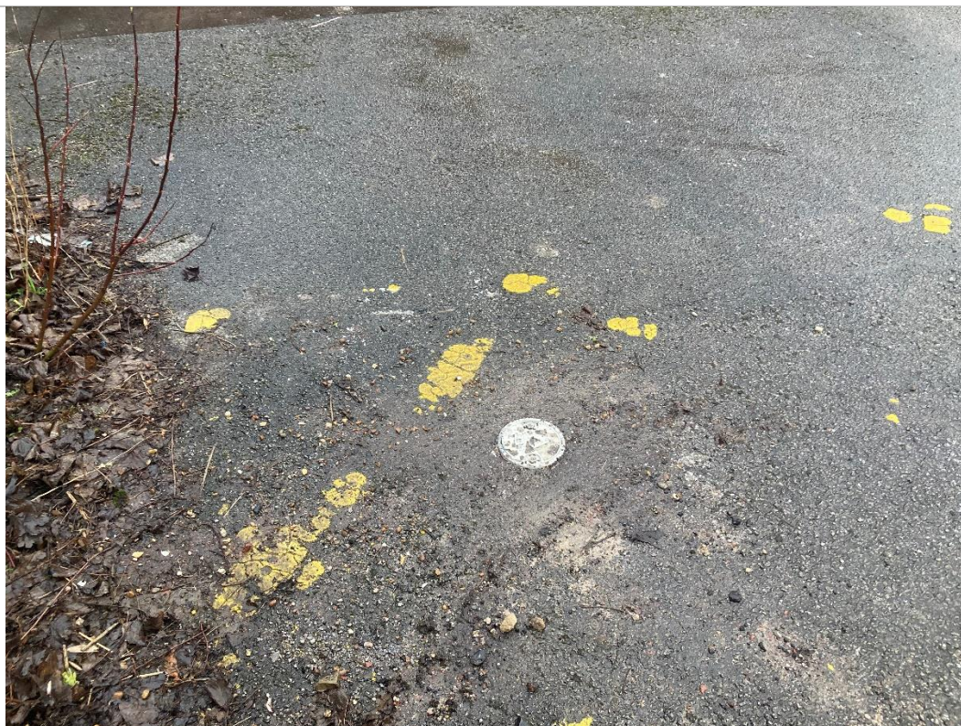
PLATE 6 WINDOW SAMPLE INSTALL CARPARK (WS103)
