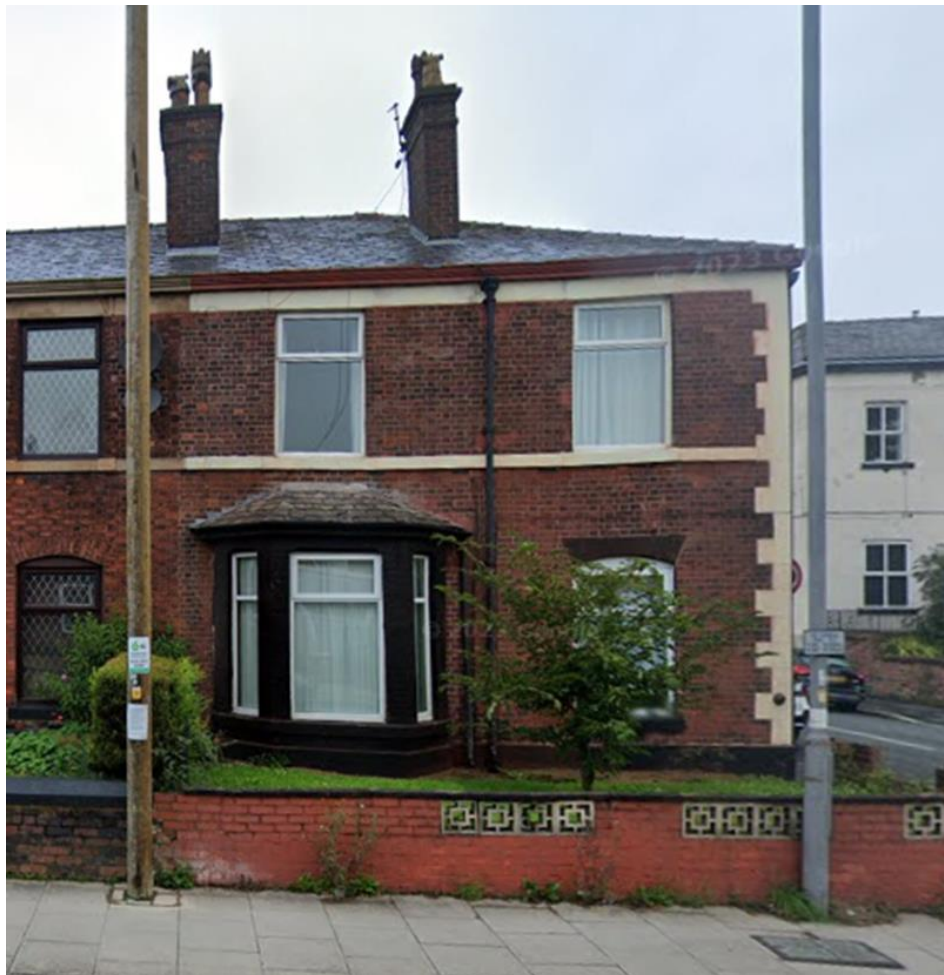
Figure 1. Front Elevation of 240 Bolton Road (Google Maps, Accessed 09/01/2025)
