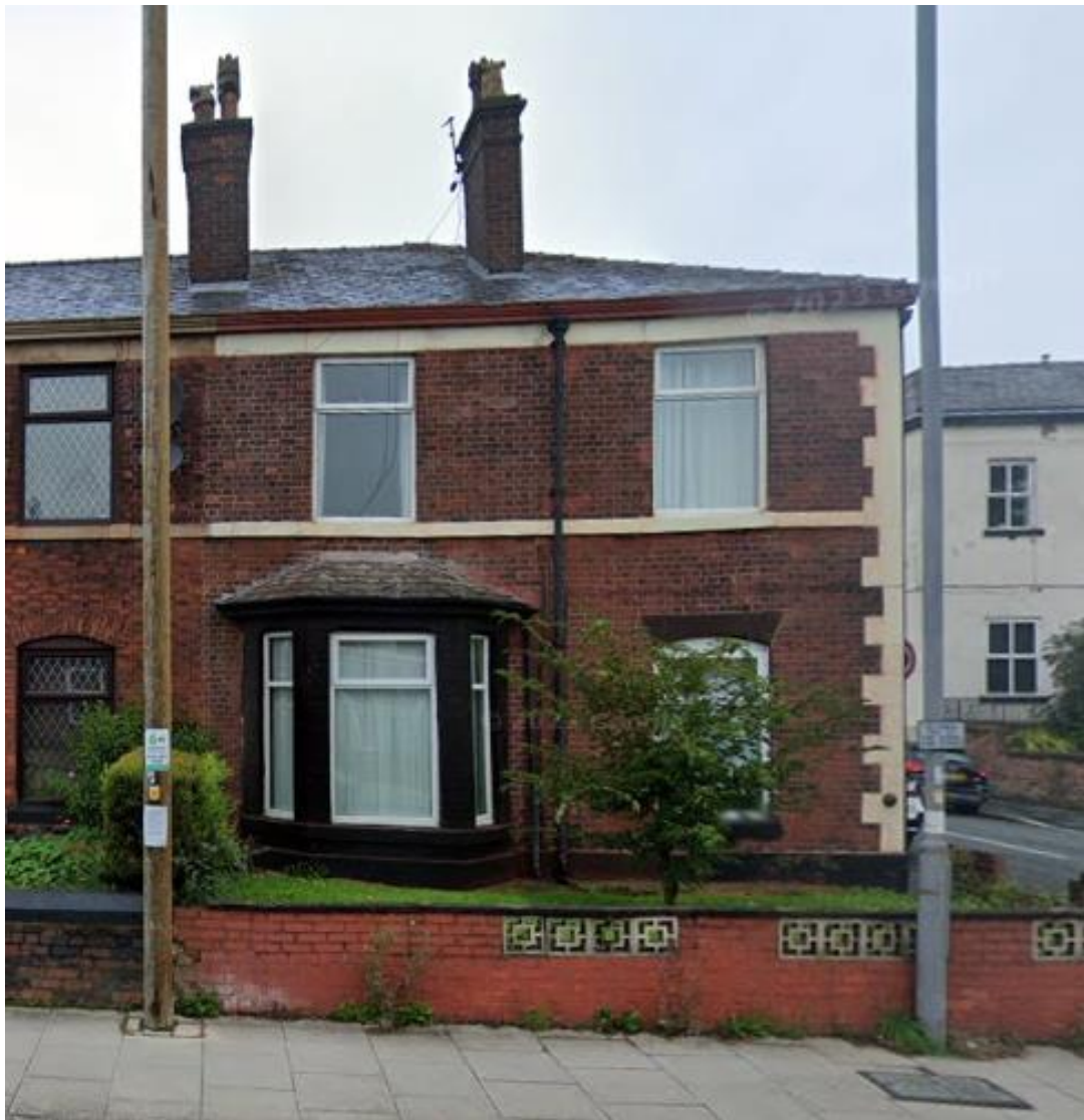
Figure 1: Front Elevation of 240 Bolton Road, Google Maps, Accessed 13/01/2025
