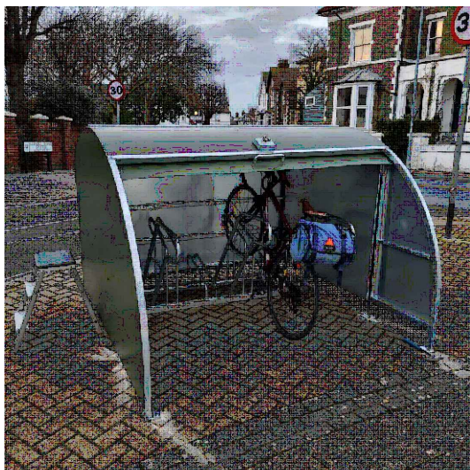
CYCLE STORAGE SHED
