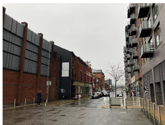
Fig 2.2: View of The Rock looking west to east.
