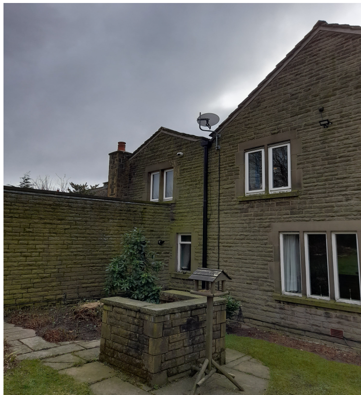
View of part northern elevation.
