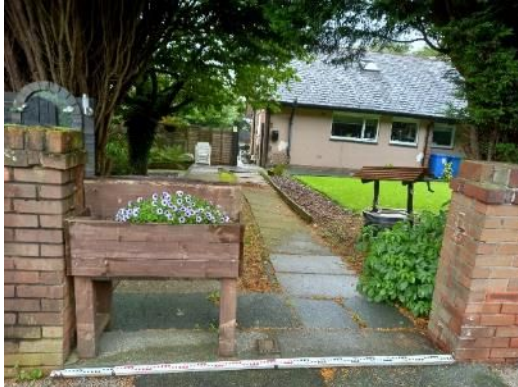
Photograph 4: View of S 3m wide site entrance. Note mature trees and crack beneath window.
