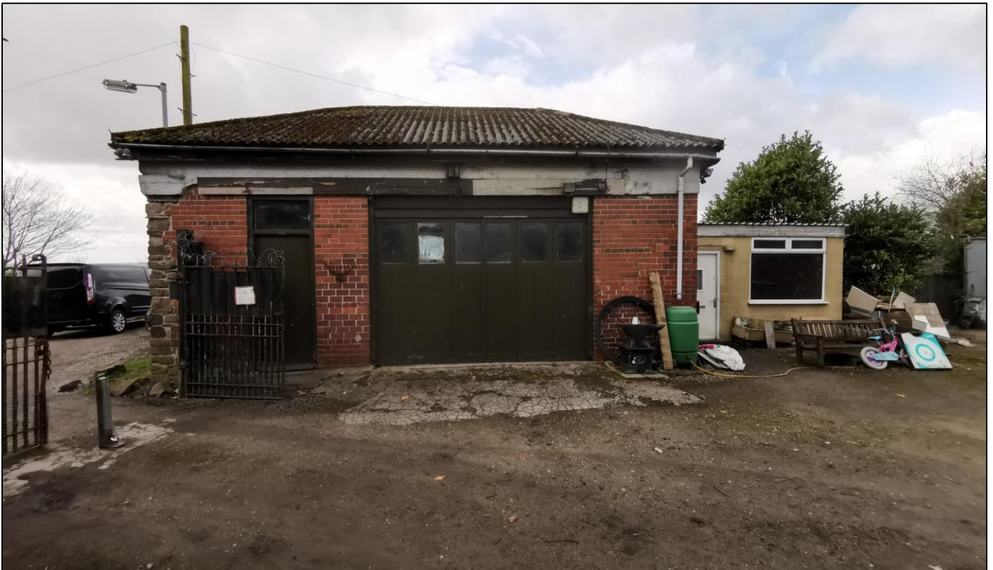
Figure 2 – View west showing 'primary elevation' of existing workshop.
