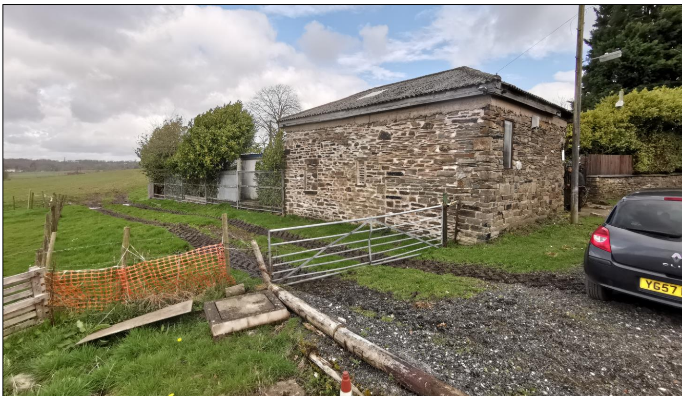
Figure 6 – View towards the northeast & workshop outside of the Site.
