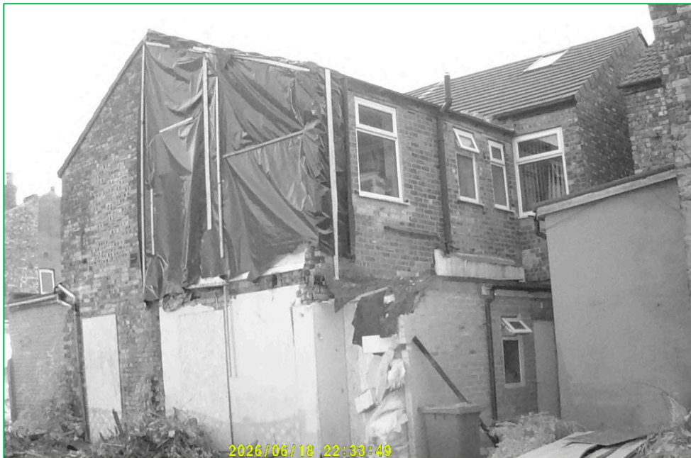
Showing the south and southeast elevation of the building using the night vision aid.
