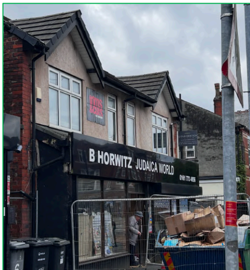
The front (north) elevation of the building
