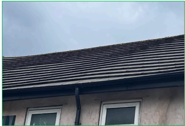
Showing the well-fitted tiles on the north elevation
