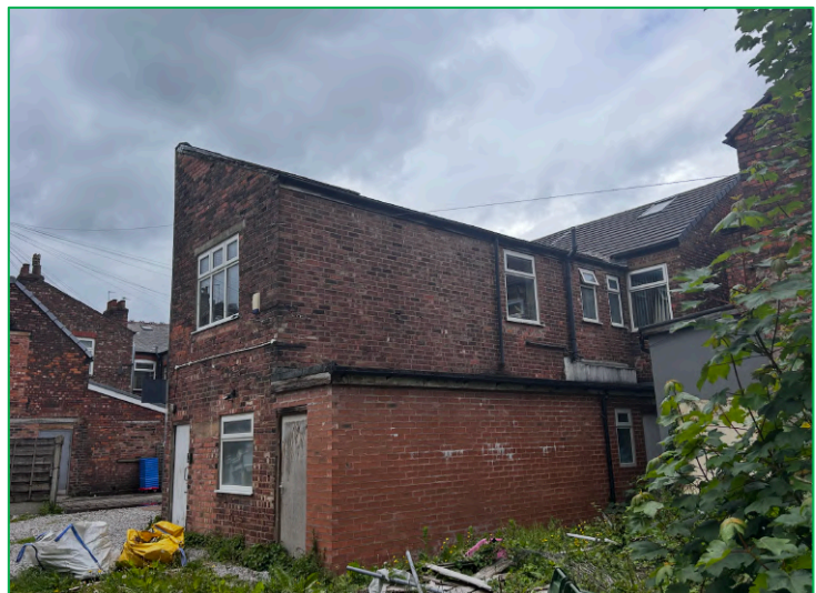
The rear (south and east) elevation of the building
