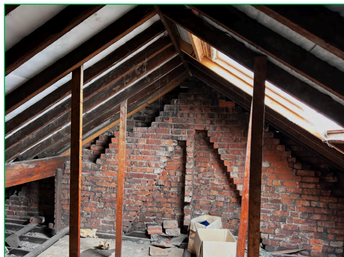
Showing the loft void, well lit by natural light
