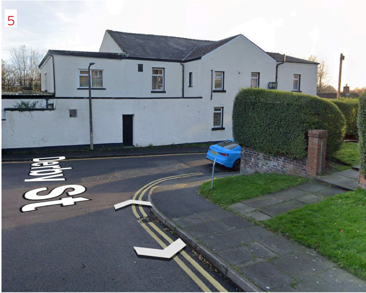
Prestwich Conservative Club opposite the application site and dedicated access to no.20 Church Lane visible
