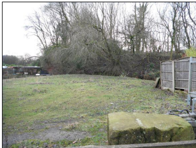
Figure 6 – Offsite landfill embankment to southeast.
