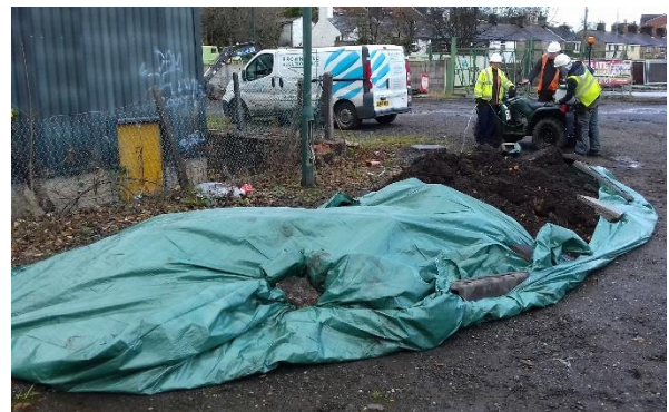
Sheeting of contaminated materials
