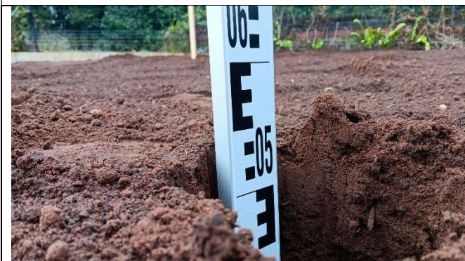
Depth measurement of pit 1 ( circa 550mm soil cover over membrane).
