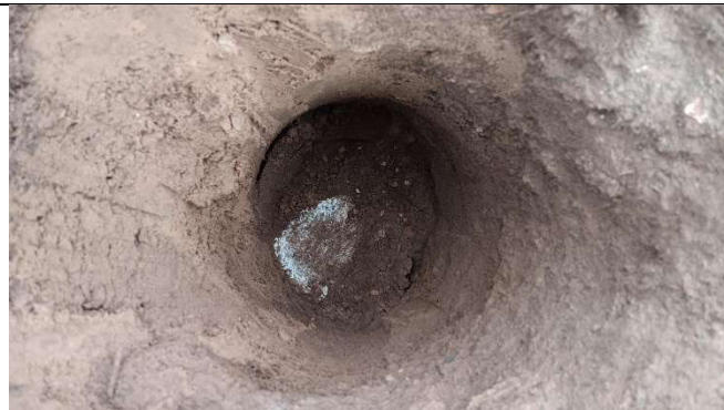
View of soil in capping layer excavation in pit 6. Demarcation membrane at base.
