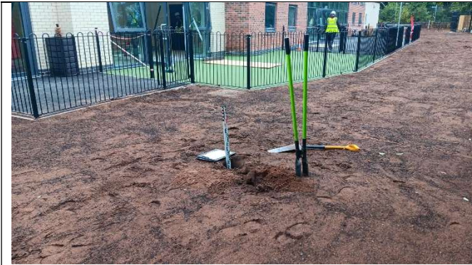
View of pit 8.
