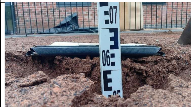
Depth measurement of pit 5 ( circa 650mm soil cover over membrane).
