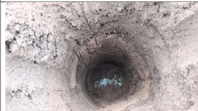
View of soil in capping layer excavation in pit 2. Demarcation membrane at base.
