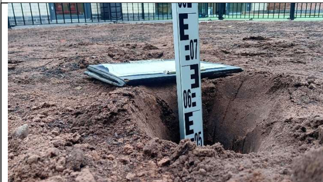
Depth measurement of pit 8 ( circa 650mm soil cover over membrane).
