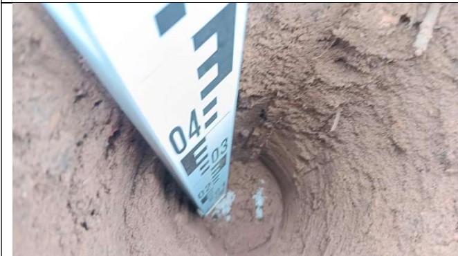
View of soil in capping layer excavation in pit 1. Demarcation membrane at base.
