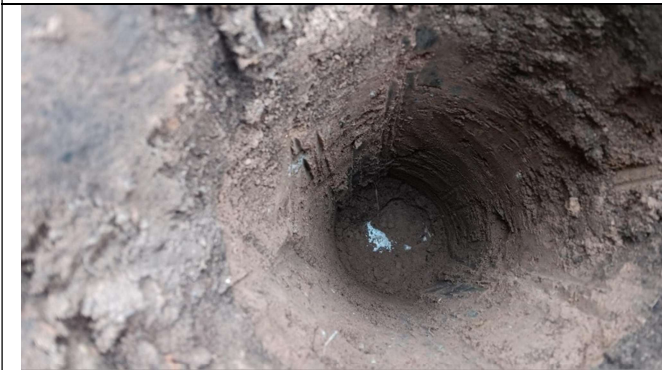
View of soil in capping layer excavation in pit 8. Demarcation membrane at base.
