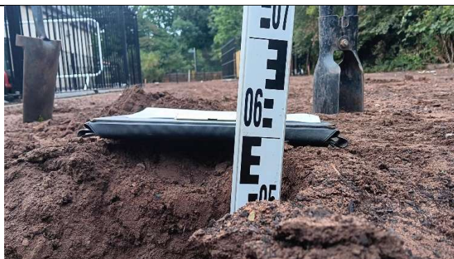
Depth measurement of pit 6 ( circa 600mm soil cover over membrane).
