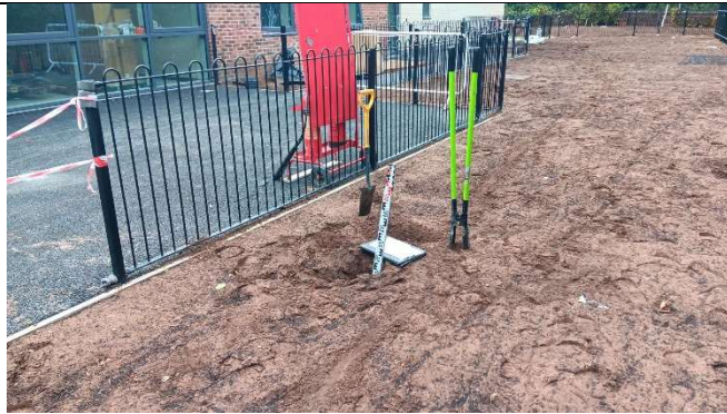
View of pit 6.
