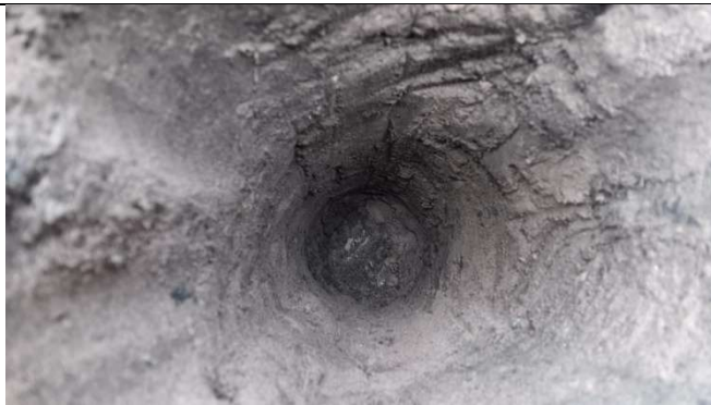
View of soil in capping layer excavation in pit 3. Demarcation membrane at base.
