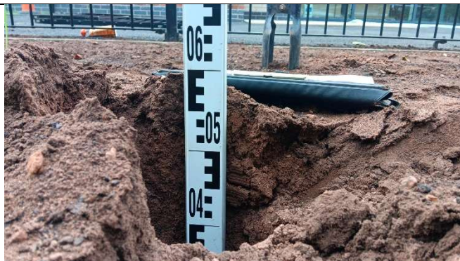
Depth measurement of pit 7 ( circa 600mm soil cover over membrane).
