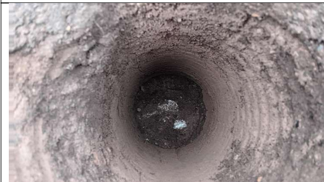
View of soil in capping layer excavation in pit 5. Demarcation membrane at base.
