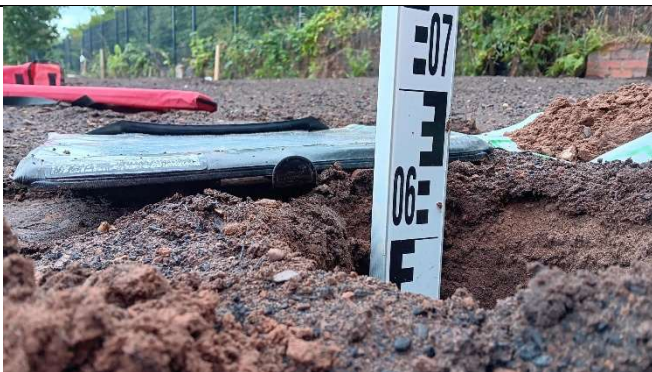
Depth measurement of pit 3 ( circa 680mm soil cover over membrane).
