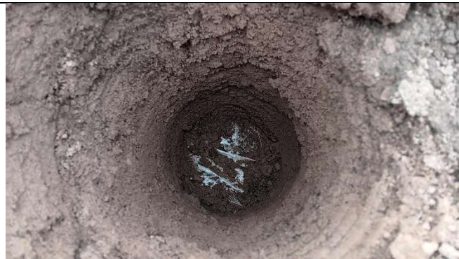
View of soil in capping layer excavation in pit 7. Demarcation membrane at base.
