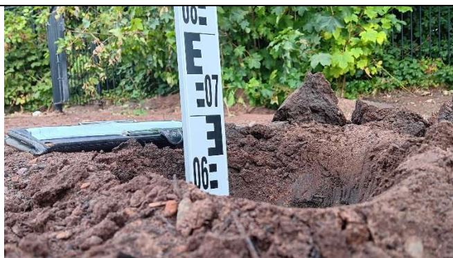
Depth measurement of pit 10 ( circa 650mm soil cover over membrane).
