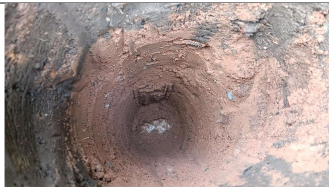
View of soil in capping layer excavation in pit 10. Demarcation membrane at base.
