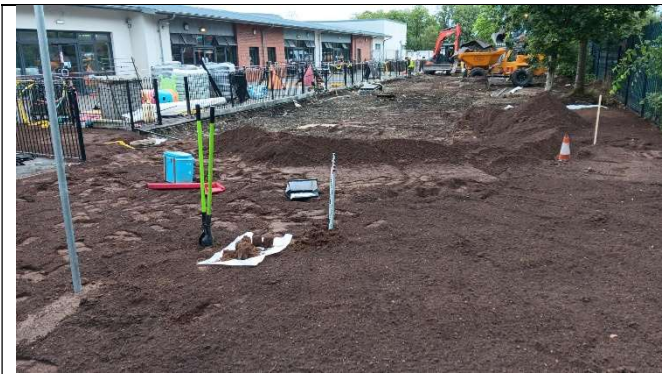
View of pit 1.
