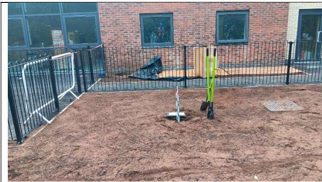
View of pit 5.
