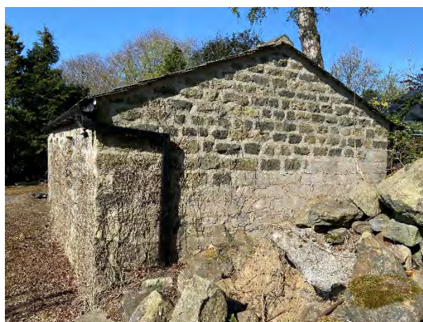
Photo 11: North-eastern gable end demonstrating stonework and mortar in good condition
