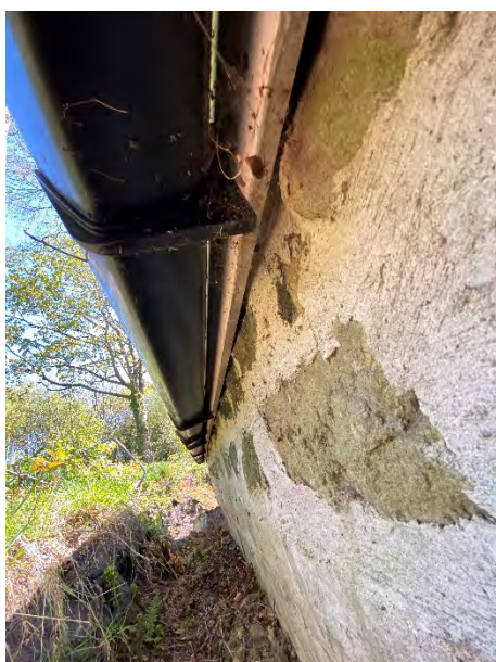
Photo 10: Partly-buried elevation of workshop
