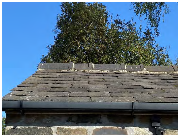
Photo 9: Slate roof tiles of building
