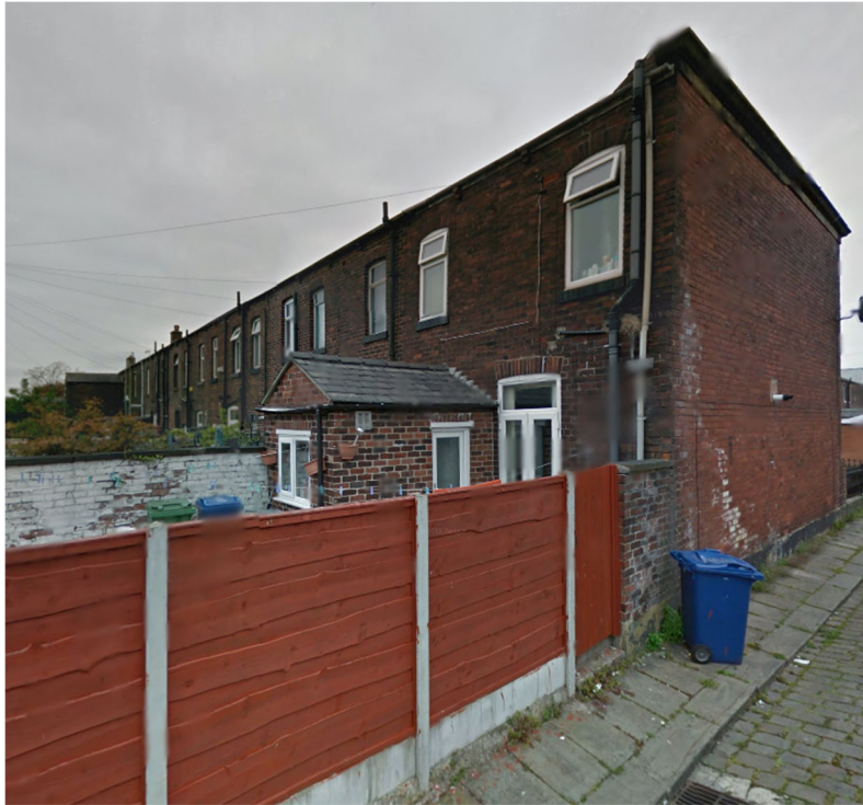
11.3 Photo taken from Google Street View of the original property pre-damage, viewing the side South Elevation, from Back Gigg Lane. Image captured May 2012.
