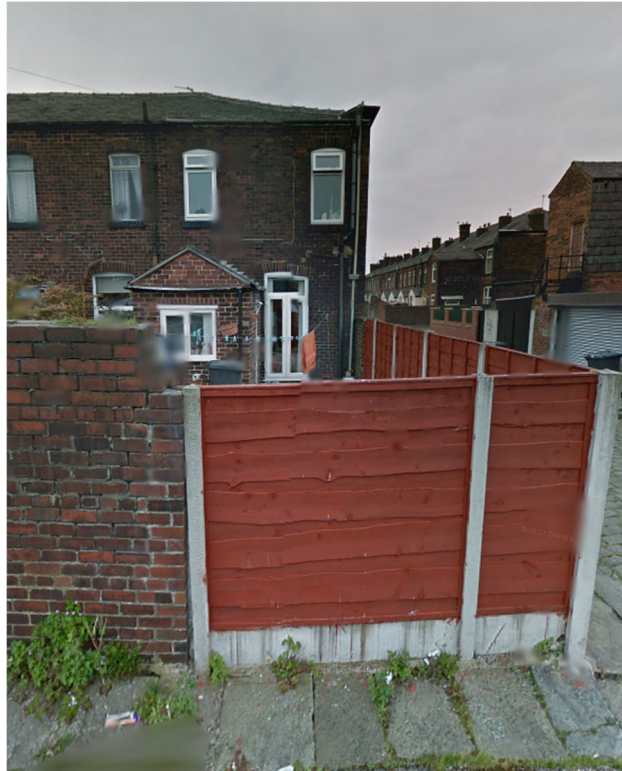
11.5 Photo taken from Google Street View of the original property pre-damage, viewing the rear East Elevation, from Back Nelson Street South. Image captured May 2012.
