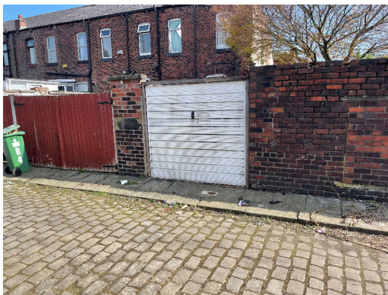
11.4 Photo taken post-damage and in its existing condition, viewing from the rear East Elevation, from Back Nelson Street South.
