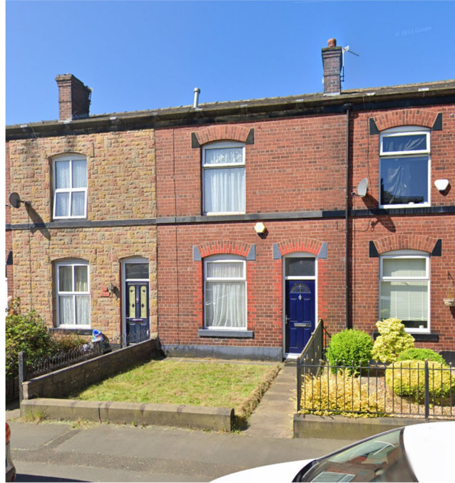
11.1 Photo taken from Google Street View of the original property pre-damage, viewing the front West Elevation, from Nelson Street. Image captured June 2023.
