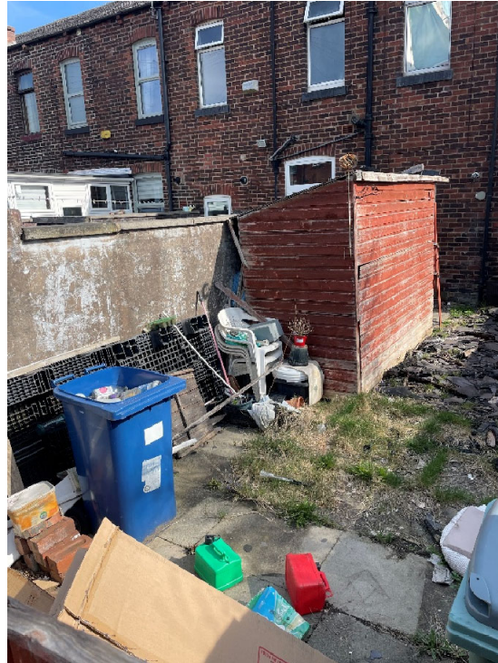
11.7 Photo taken post-damage and in its existing condition, from rear East Elevation.
