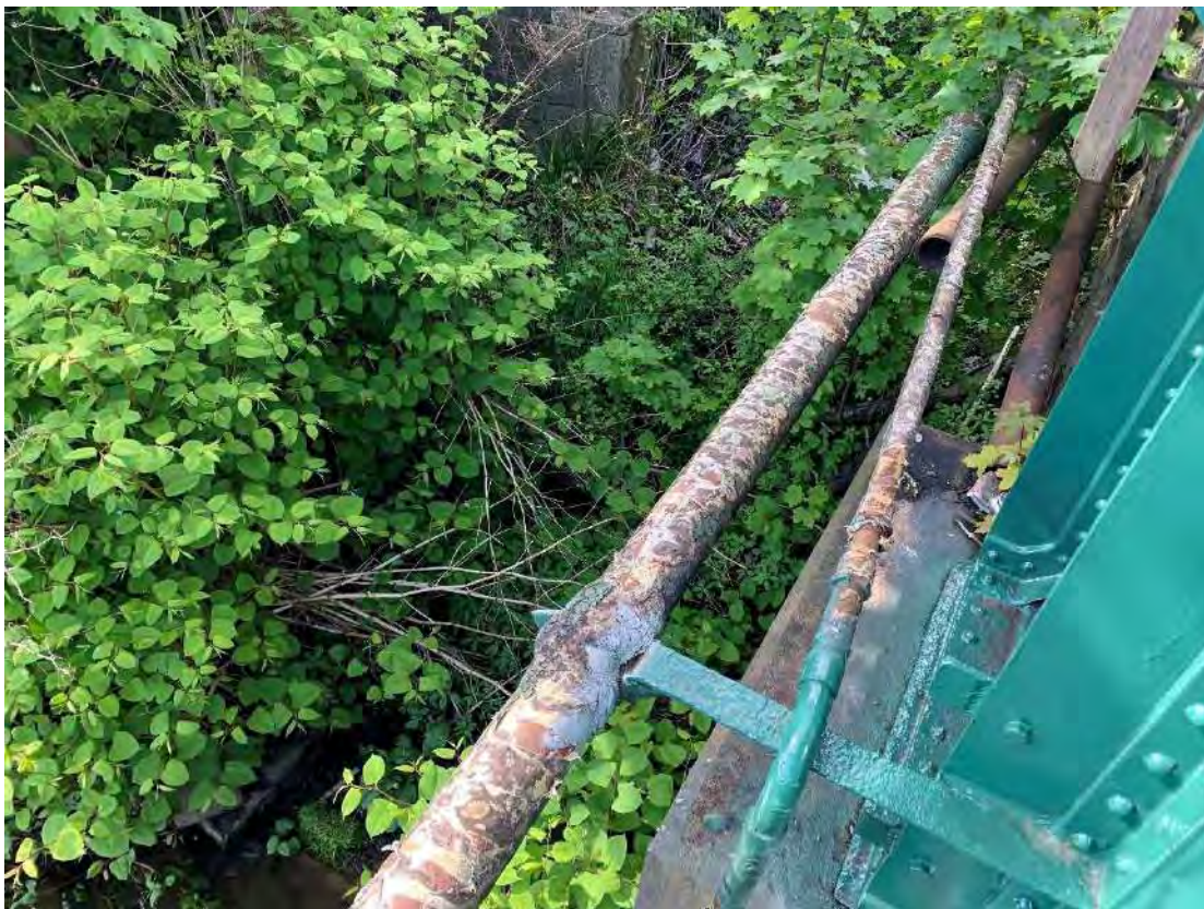
17 – Outfall to River Irwell
