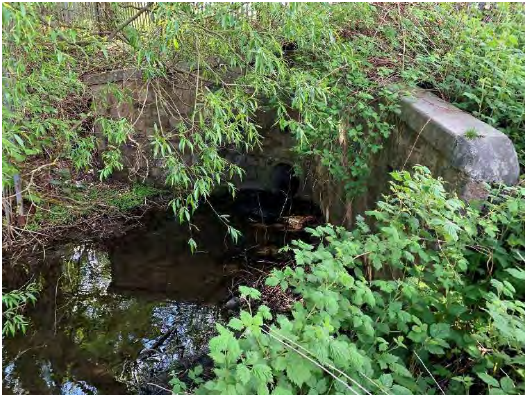
6 – Pipe Outlet to stream
