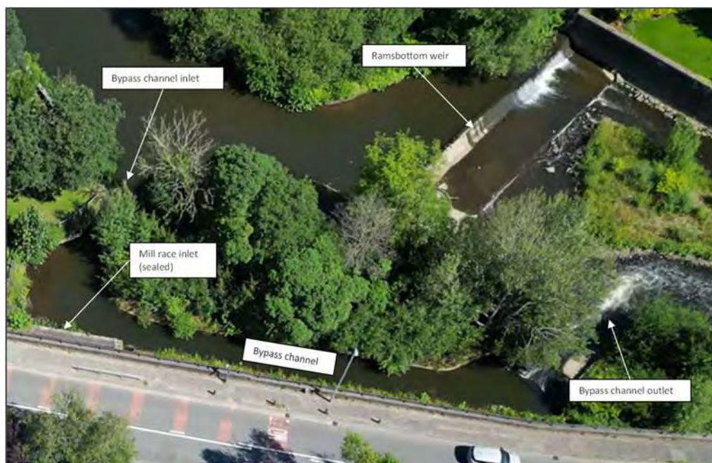
Figure 6: River Irwell Immediately Upstream of Bridge Street/Peel Bridge (Drone Footage taken on 7 July 2023)
