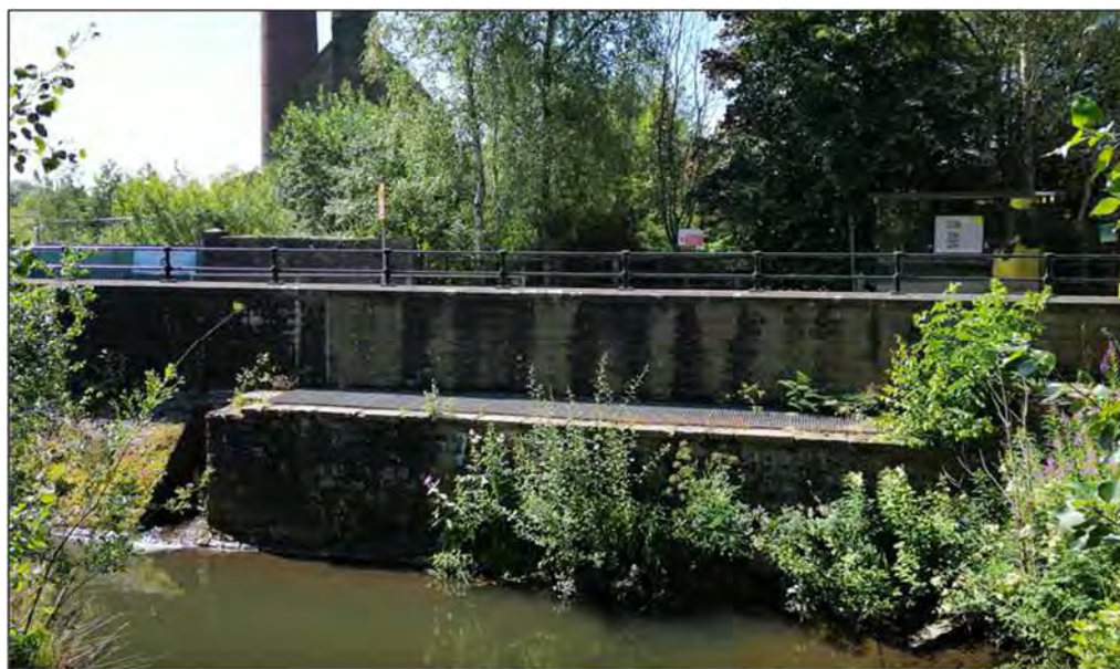
Figure 8: Mill Race Inlet (Now Sealed) (Looking South)
