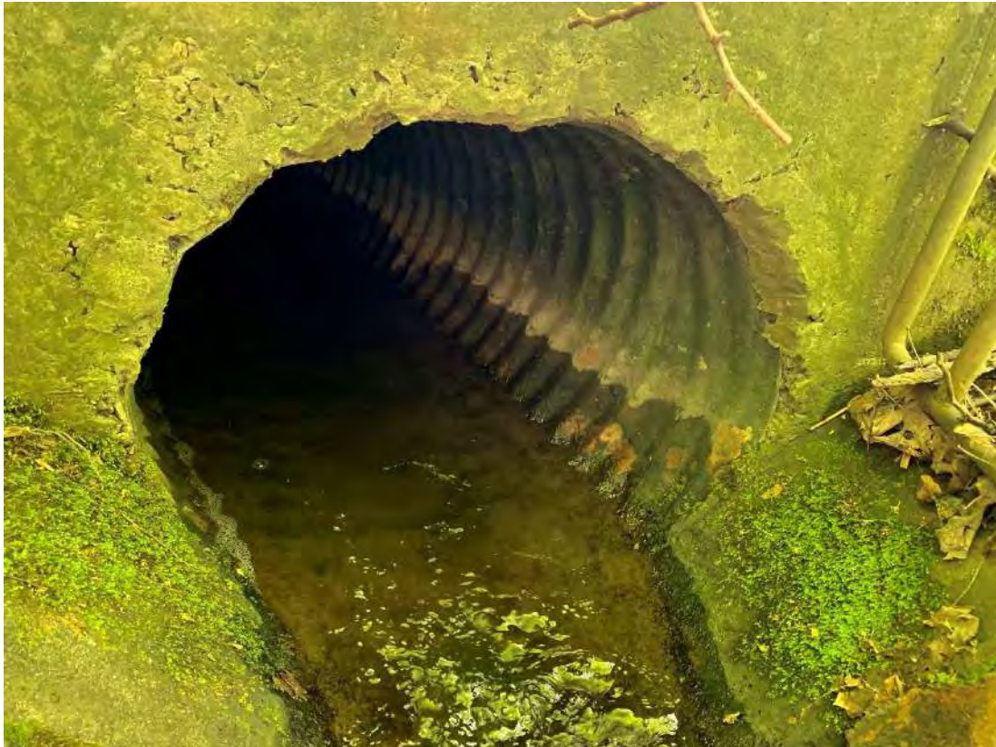
14 – Pipe inlet beneath railway embankment (taken through grill)
