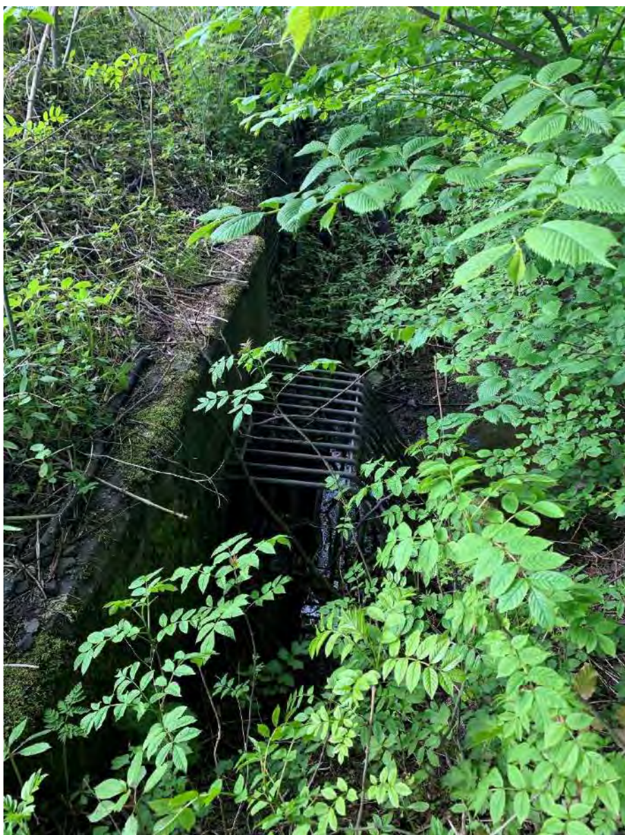
13 – Grill to pipe inlet beneath railway embankment
