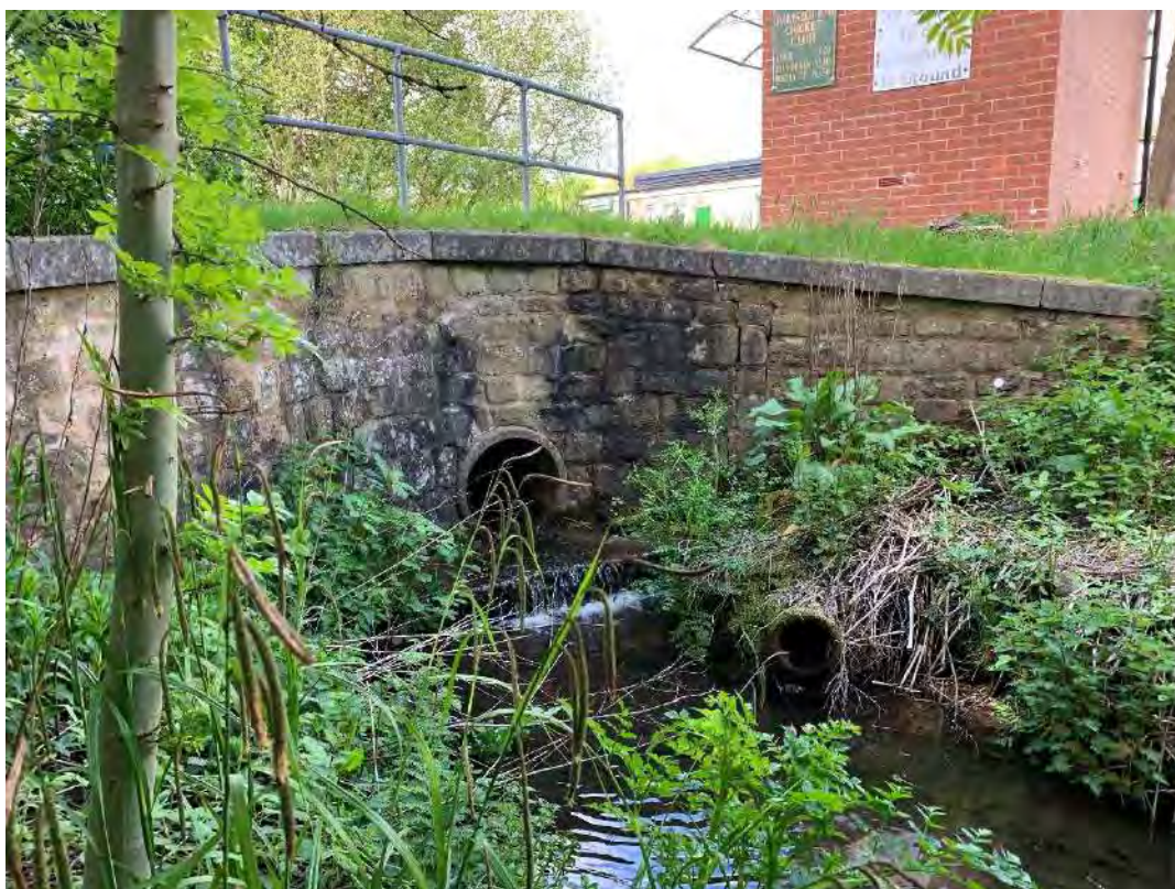
9 – Downstream Pipe / headwall beneath Cricket Club access road
