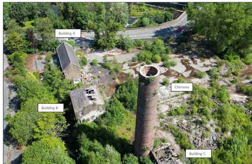
Figure 5: View of Existing Buildings (Drone Footage taken on 7 July 2023)
