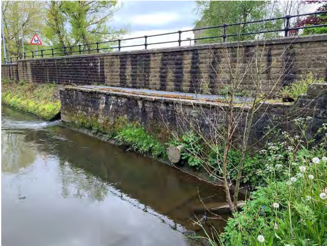
1 – Blanked off pipe inlet
