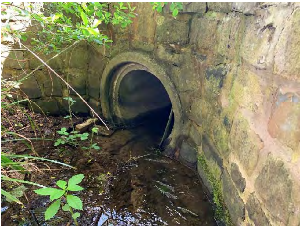
8 – Upstream Pipe / headwall beneath Cricket Club access road
