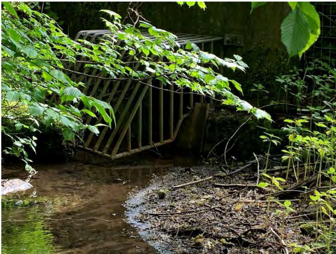
12 – Grill to pipe inlet beneath railway embankment
