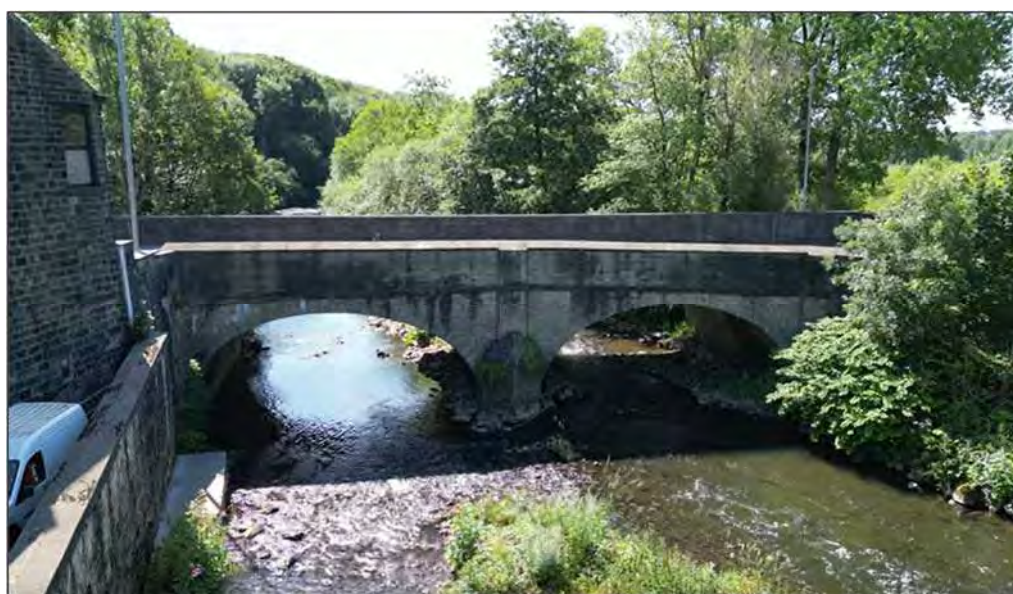
Figure 7: Peel Bridge Looking Downstream (South)
